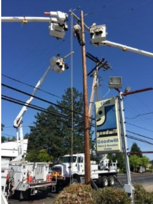
Installing fiber along North State Street
