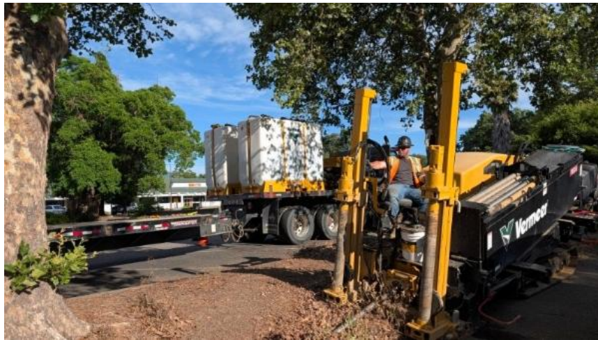
Ukiah Gigabit Fiber project in construction
