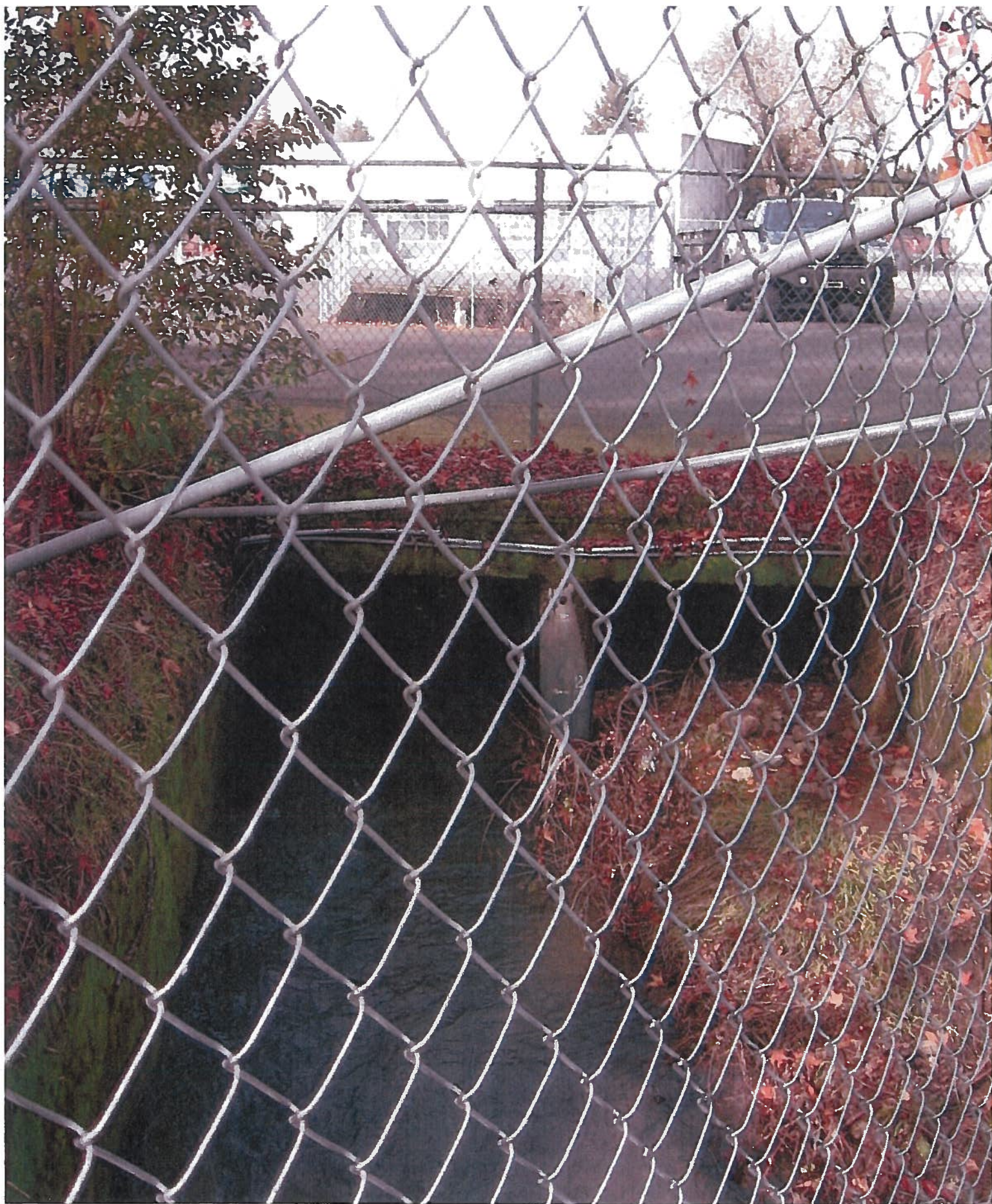
Gibson Creek between Mason/Main St., 1/2016
