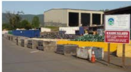
Ukiah Transfer Station
