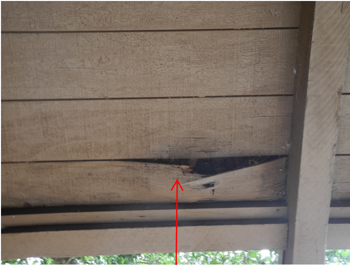
damaged decking
