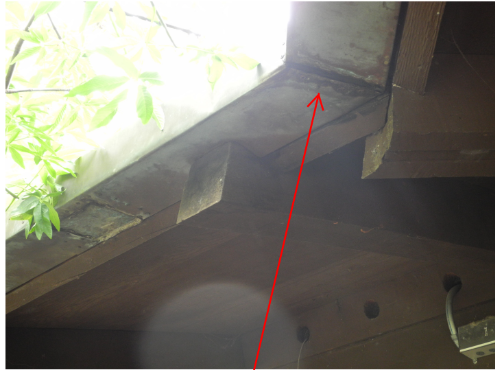
leaking gutters
