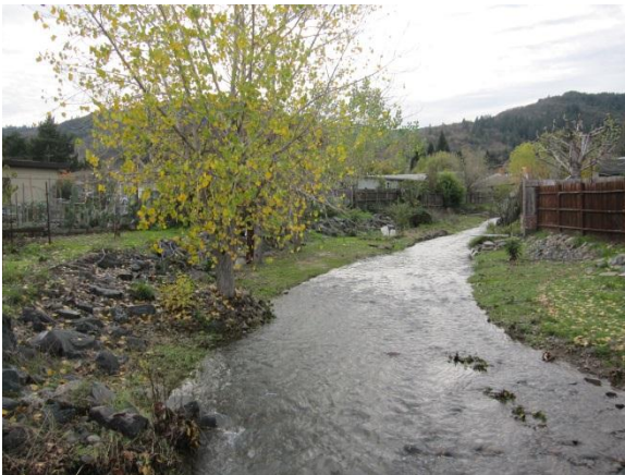
Mulberry Street culvert – after a storm – looking west
