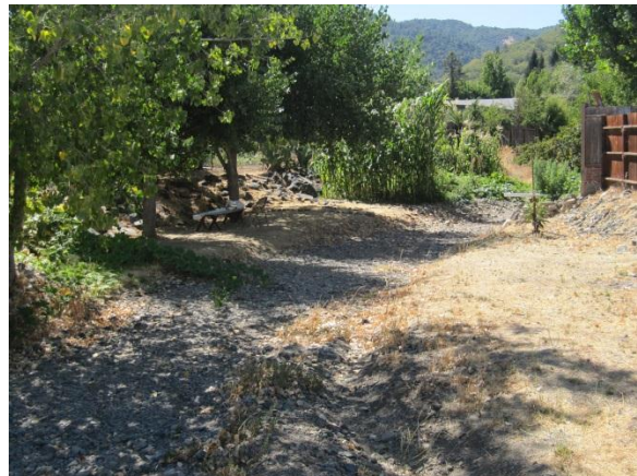
Mulberry Street culvert – in dry period – looking west
