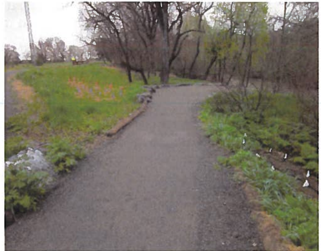
SHN provided construction staking, materials testing, and daily field inspection during construction of the half mile long Riverside Park Trail.
