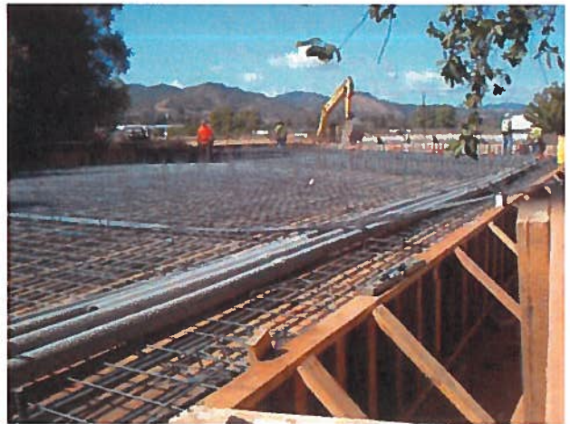
SHN provided Resident Engineering, Environmental Engineering and Construction Inspection Services for the construction of the Orchard Avenue Bridge. The Project was completed ahead of schedule and below the estimated construction management budget.
