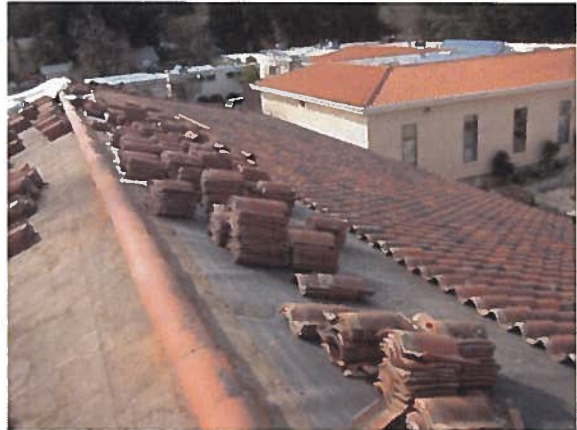
SHN provided construction management and material testing services for the Civic Center Roof Rehabilitation, Skate Park, and Anton Stadium Repair projects. SHN has a proven track record of working successfully with the City of Ukiah
