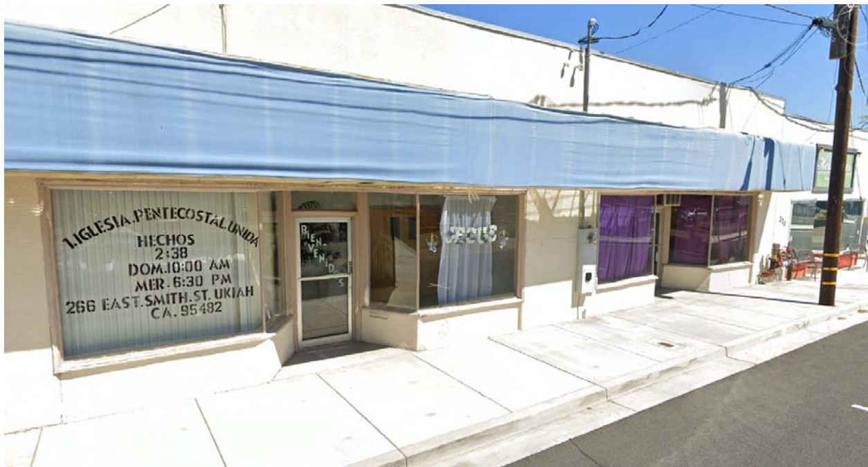
Figure 3. Iglesia Pentecostal United Church located on the project parcel
