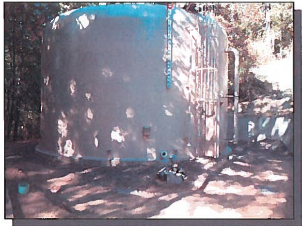
Phillipsville Community Service District's new water reservoir, after repainting.
