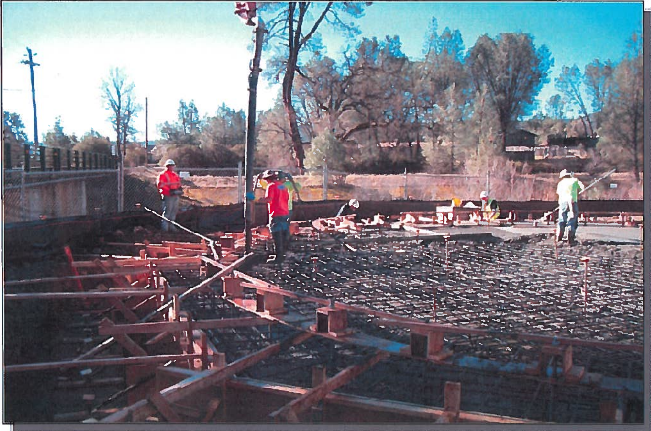
Water tank foundation concrete placement activities for the Spring Valley Water Improvement project.
