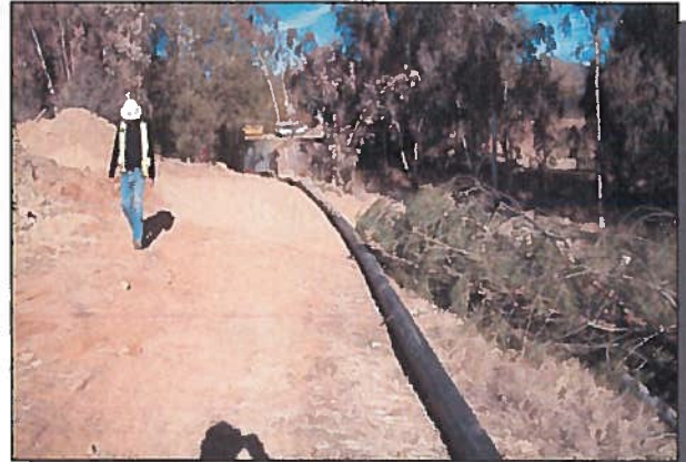
Welded HDPE water main pipe to be installed underneath Highway 29 for the Bell Hill Road project.
