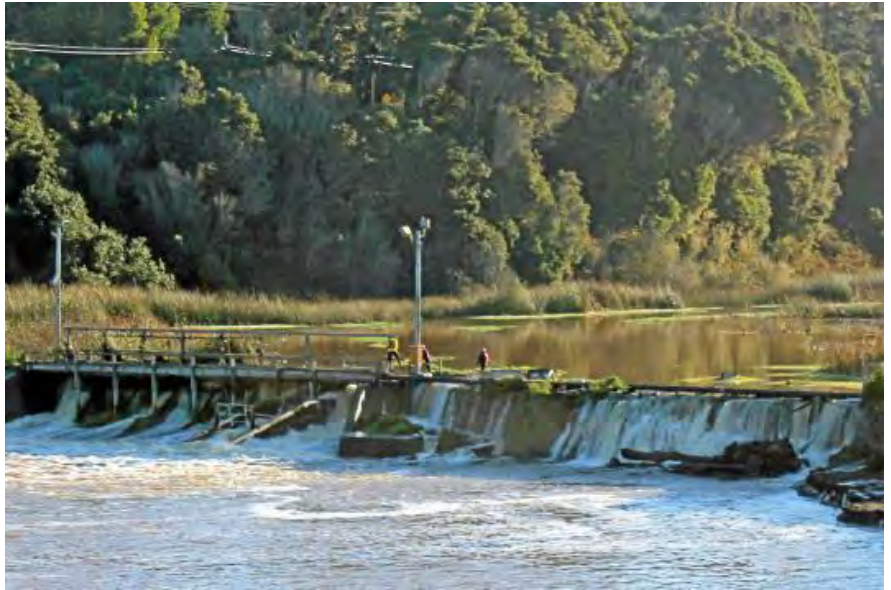
Figure 4-12: Pudding Creek Dam Overflow
