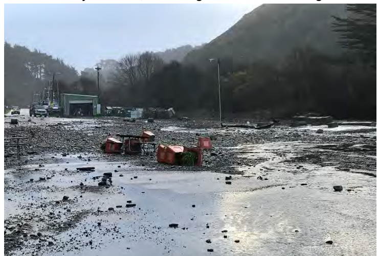
Figure 3-2: Damage to Arena Cover Parking Lot in 2017
