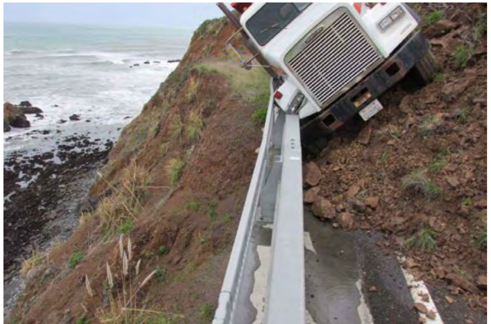
Figure 4-44: Mudslide on Highway 1 in Mendocino County
