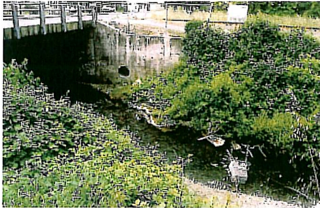
Orrs Creek at the Ford Street Bridge
