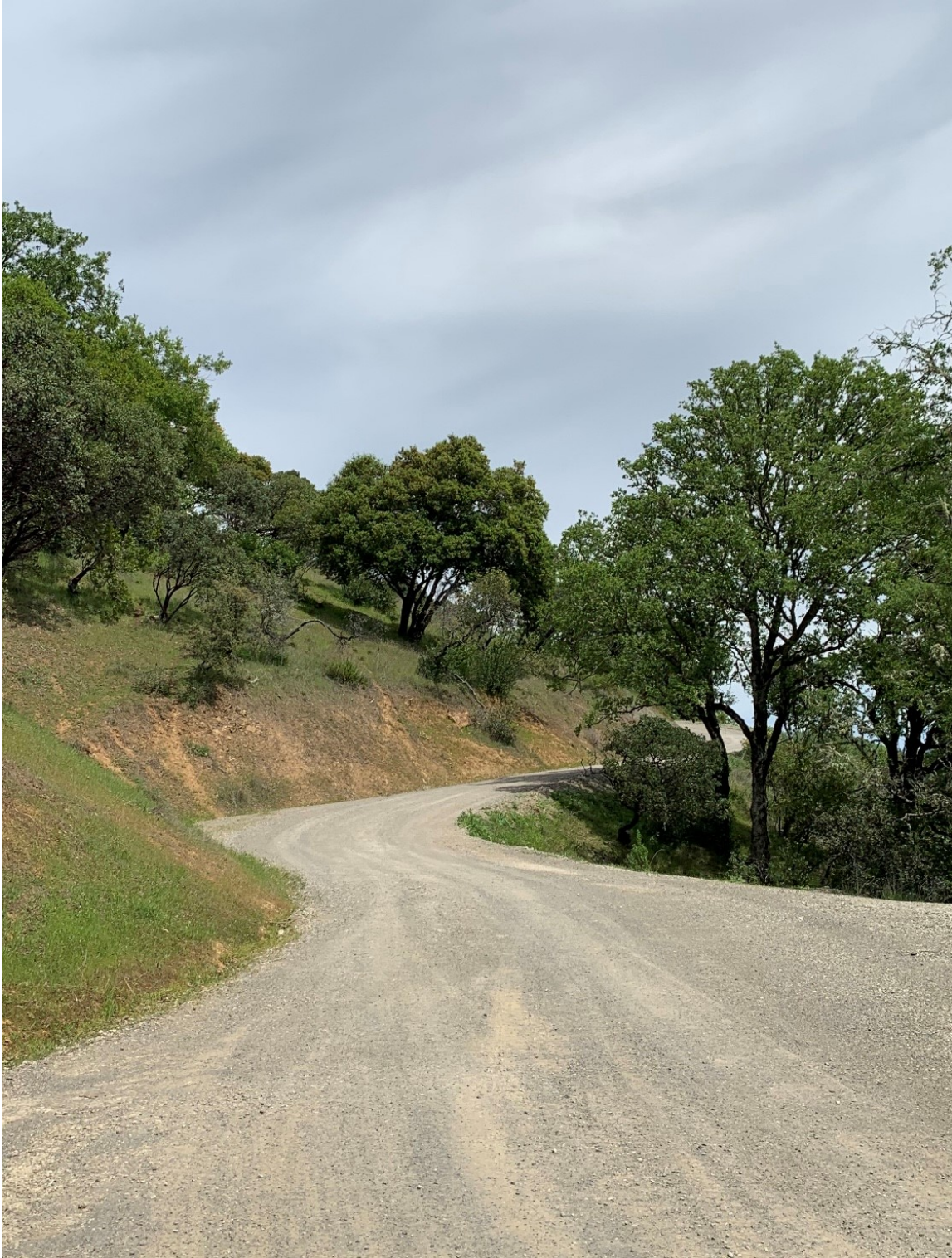
Existing access road
