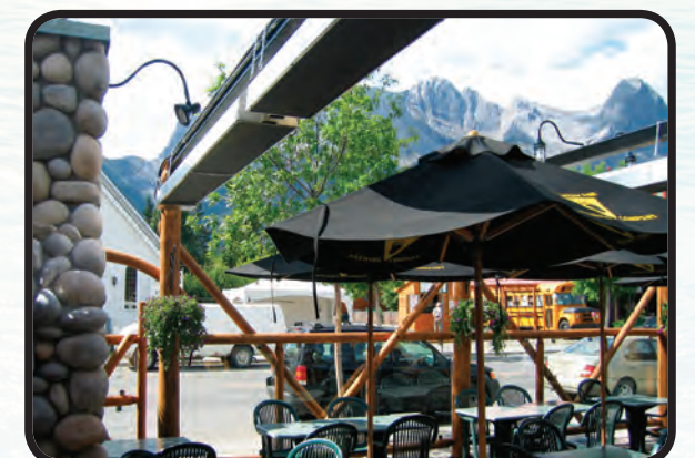
LOW CLEARANCE TO COMBUSTIBLES
