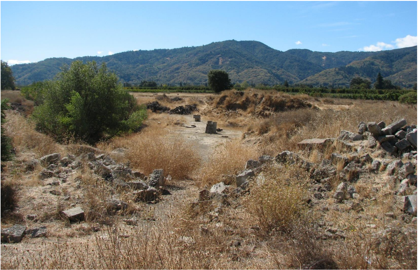
Remnant Pit, Debris Piles and berms impeding the floodway, photographed in October
