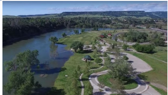
Riverbend Park Flood Damage Restoration 2017 CSDA Innovative Program/Project of the Year
