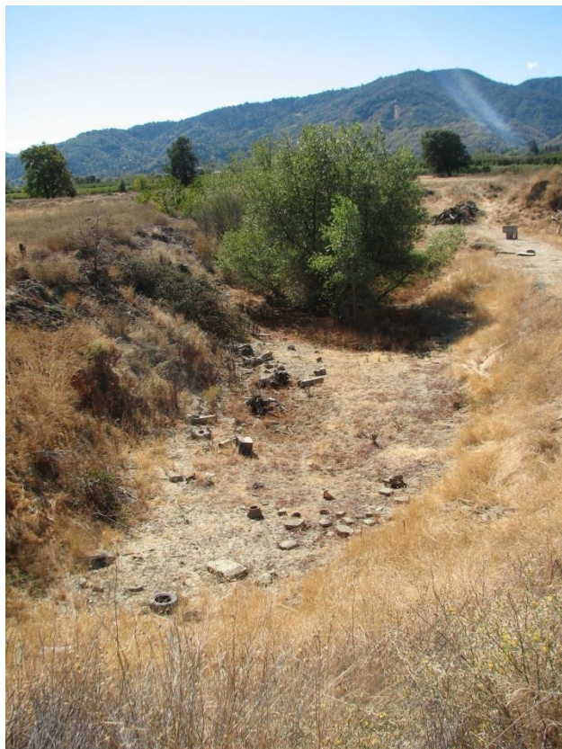
Remnant Pit of former sewer treatment plant photographed in October, dry conditions
