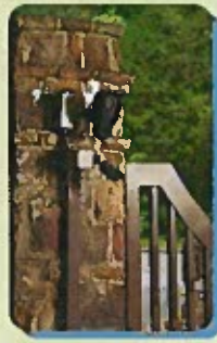
Electric & Existing Structure / Pole
