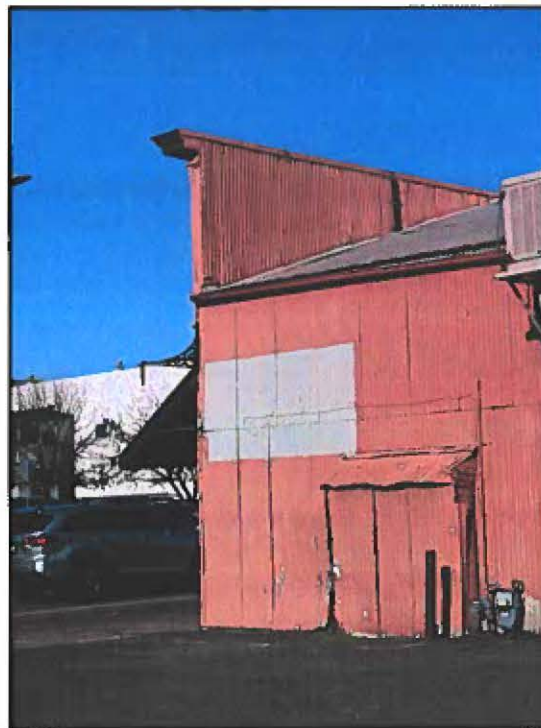
Photo 39: West elevation false front (looking NW)
