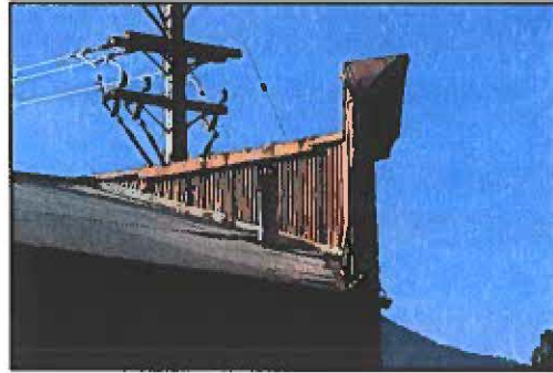
Northwest corner, False Front Detail
