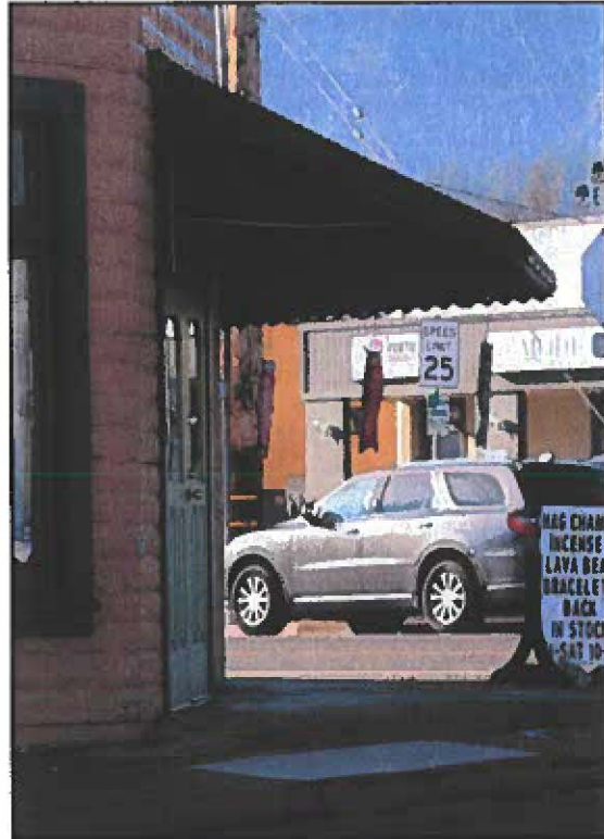
Photo 32: Northwest corner, detail of metal awning
