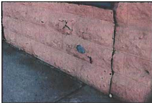
West Elevation, Pressed Tin Detail
