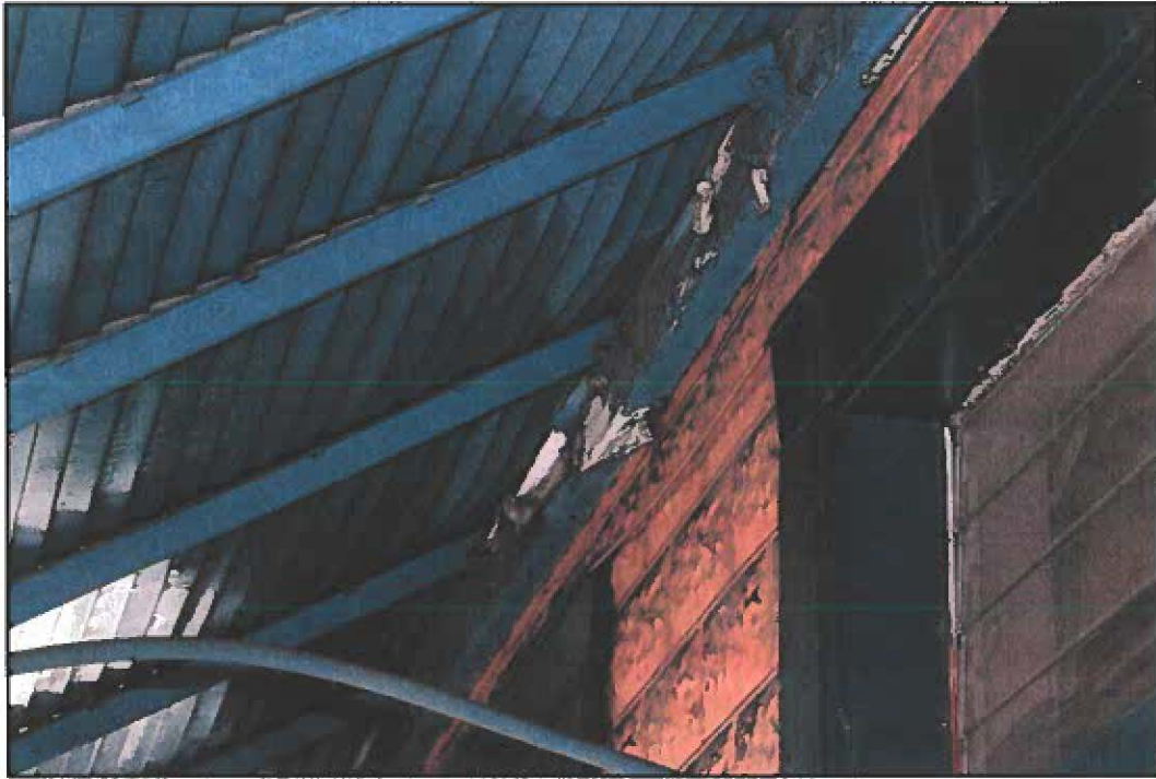
Photo 36: West elevation, ceiling of awning
