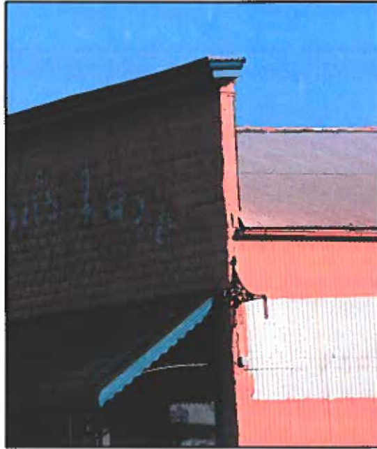
Photo 38: West elevation, false fronting (looking NE)
