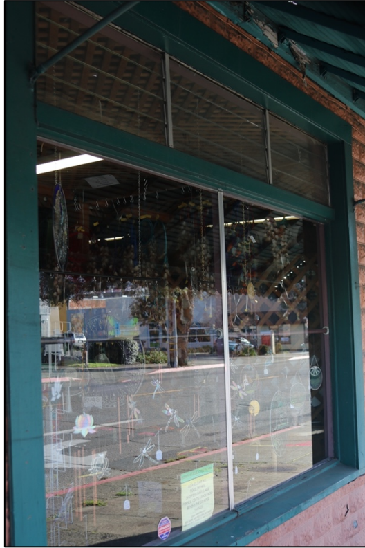
Photo 33: West elevation, middle window with jalousie transom (ca 1963)
