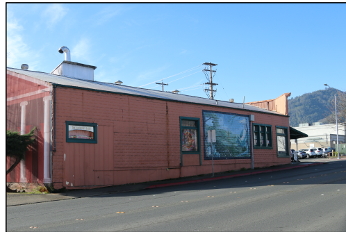
North Elevation (Perkins Street)
