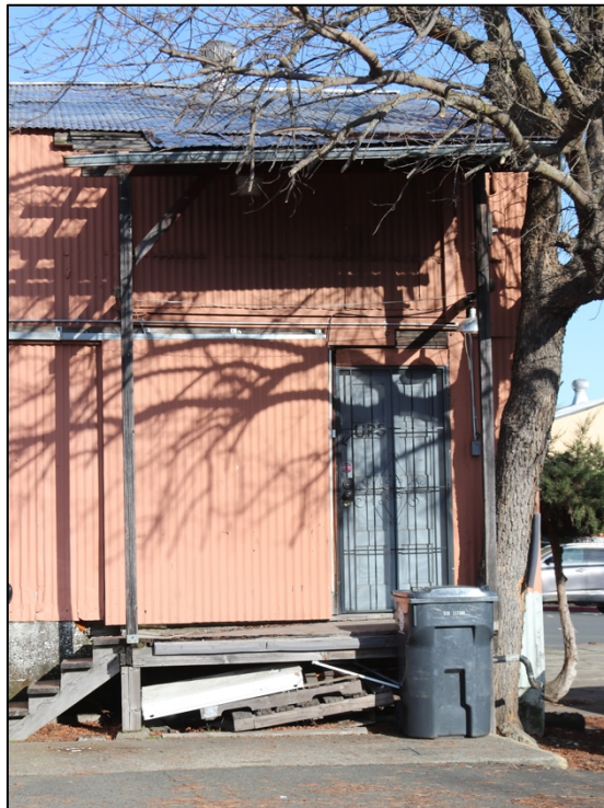
Photo 42: South elevation, pedestrian entrance at SE corner
