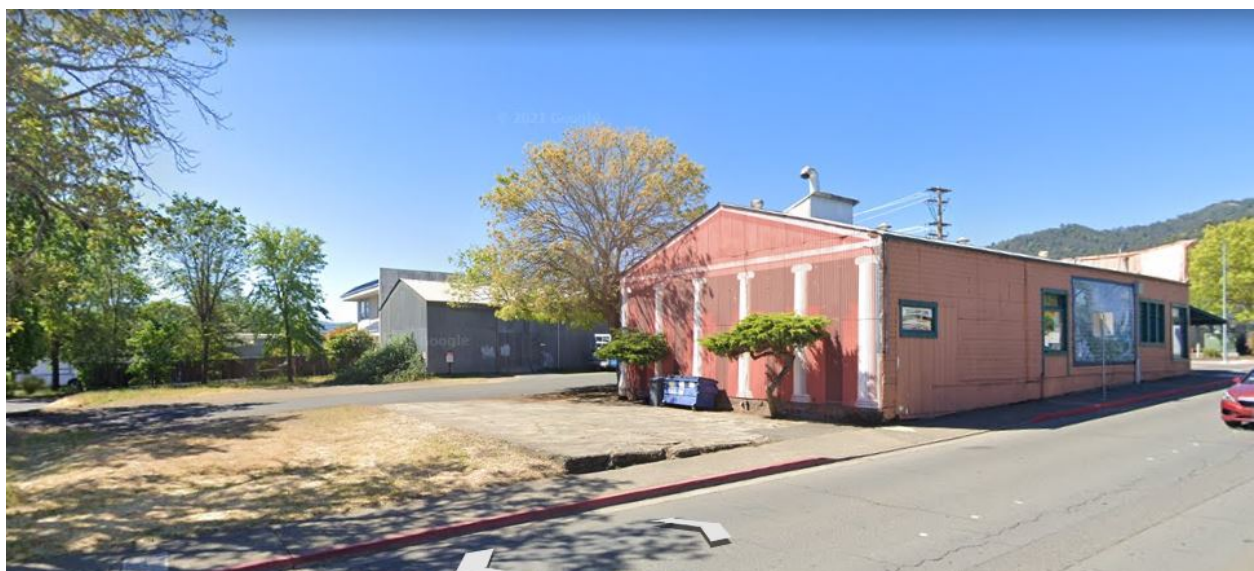
Existing Buildings looking west from Perkins Street
