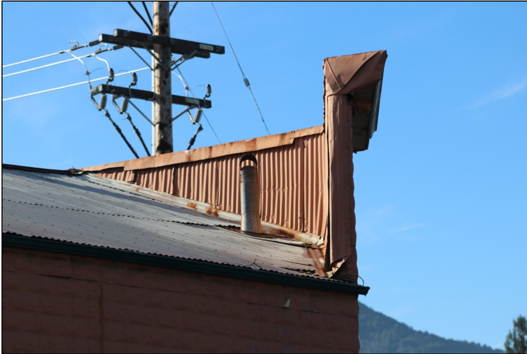
Photo 39: West elevation, false front (looking SW)
