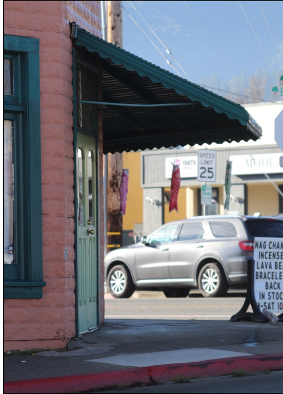
Photo 31: Northwest corner, detail of metal awning
