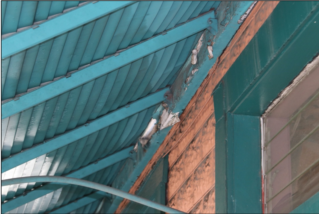
Photo 35: West elevation, ceiling of awning
