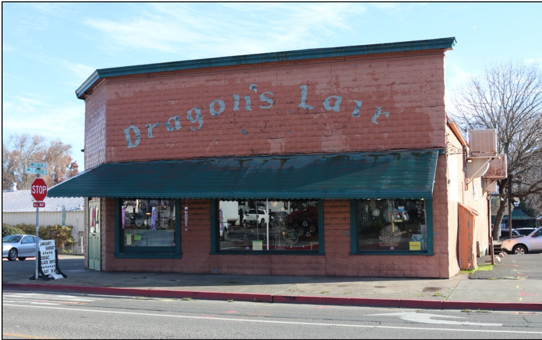
Photo 27: West elevation (facing South Main Street)
