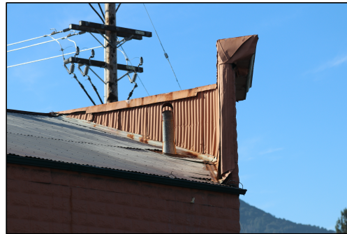
Northwest corner, False Front Detail
