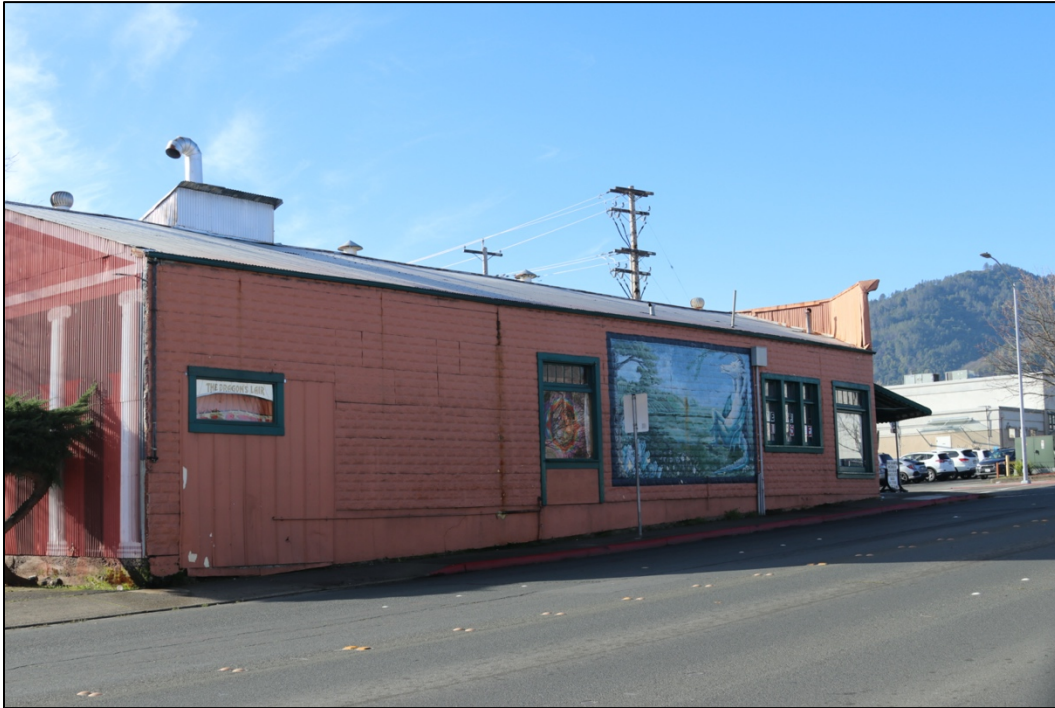
Photo 45: North elevation (fronting Perkins Street)
