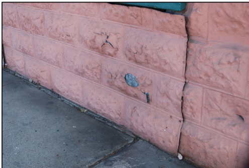
West Elevation, Pressed Tin Detail
