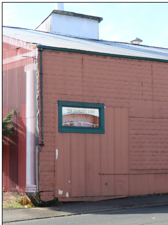
Photo 46: North elevation, infilled bay at NE corner
