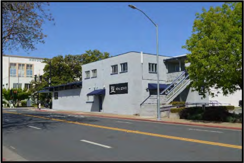
Side/South & Rear/East Elevations
