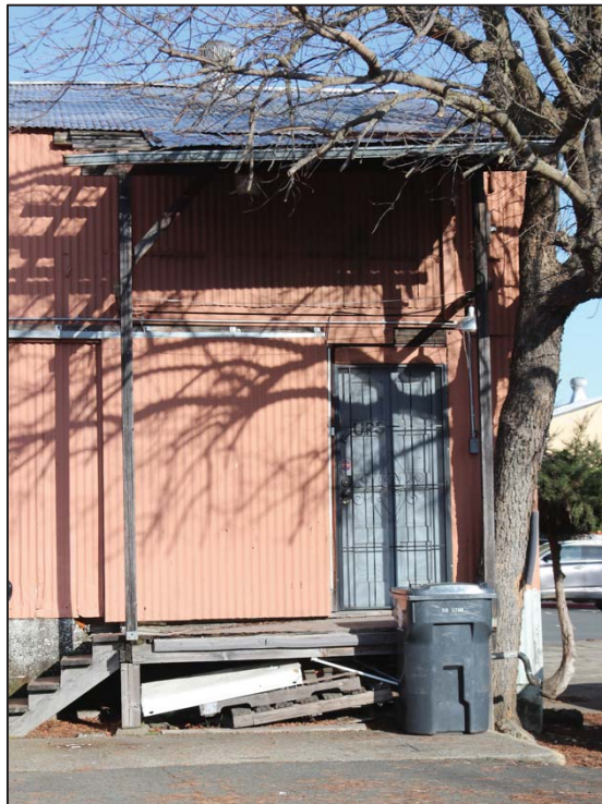
Photo 42: South elevation, pedestrian entrance at SE corner
