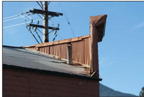
Northwest corner, False Front Detail
