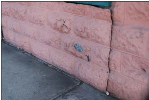
West Elevation, Pressed Tin Detail
