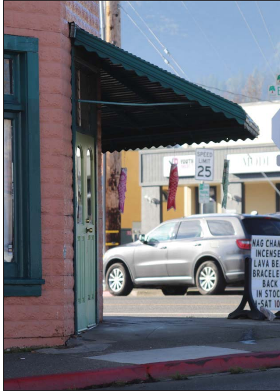
Photo 31: Northwest corner, detail of metal awning
