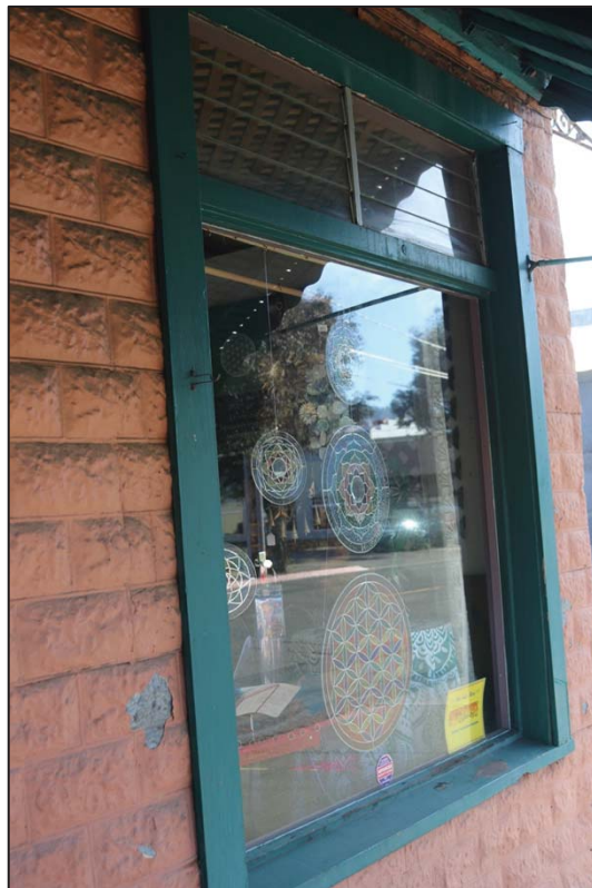
Photo 34: West elevation, south window with jalousie transom (ca 1963)
