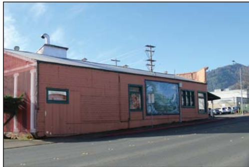
North Elevation (Perkins Street)
