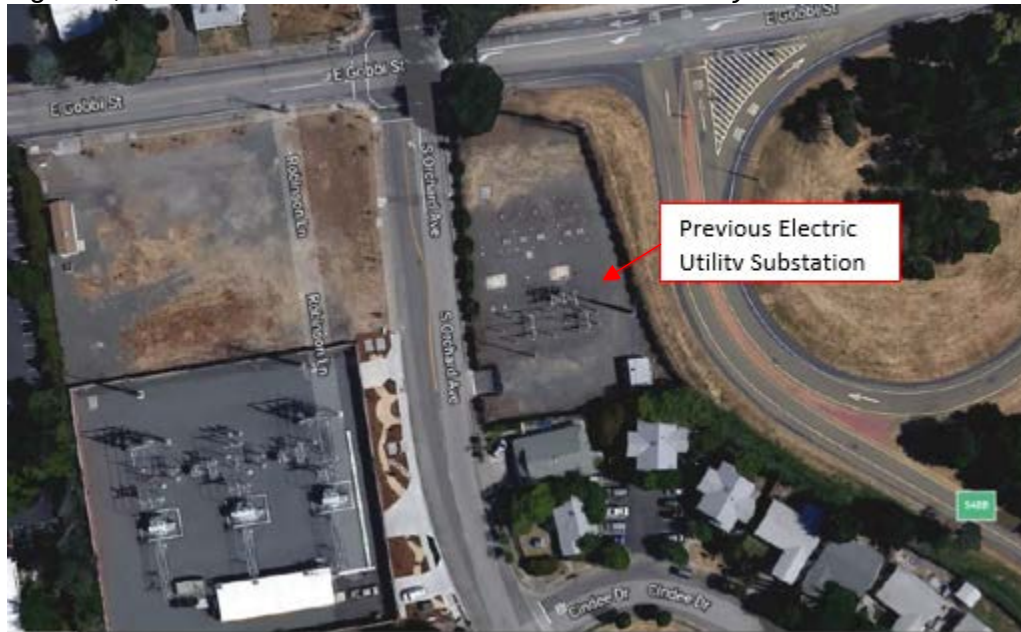
Figure 1, Aerial Photo of Site with Previous Electric Utility Substation
