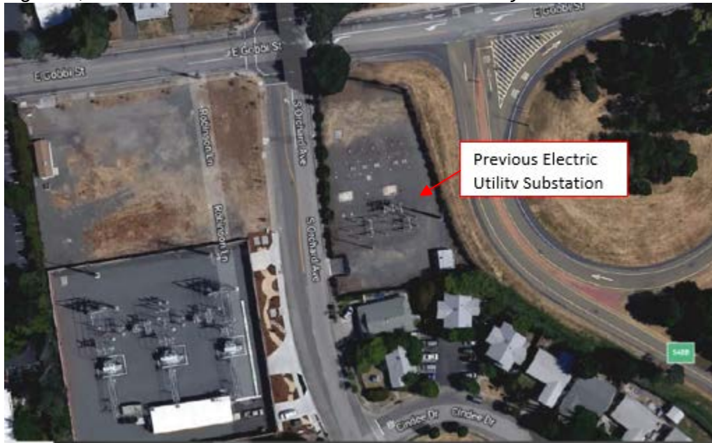
Figure 1, Aerial Photo of Site with Previous Electric Utility Substation
