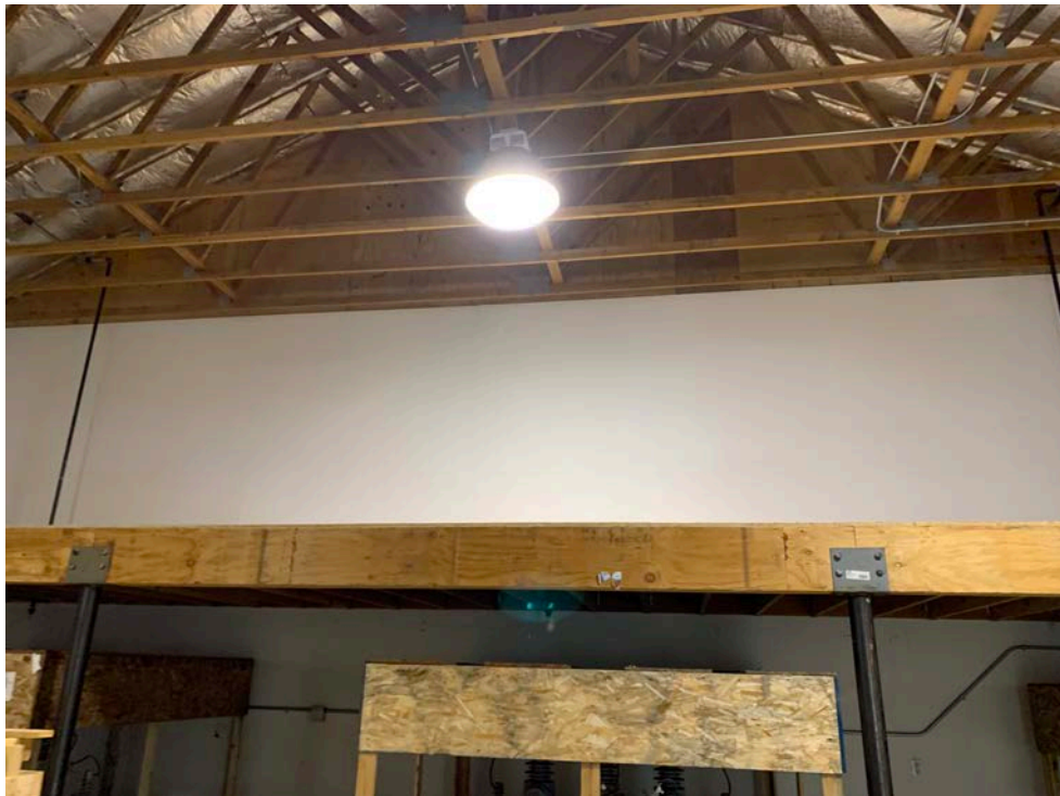
5 EXISTING BAY 2 MEZZANINE
