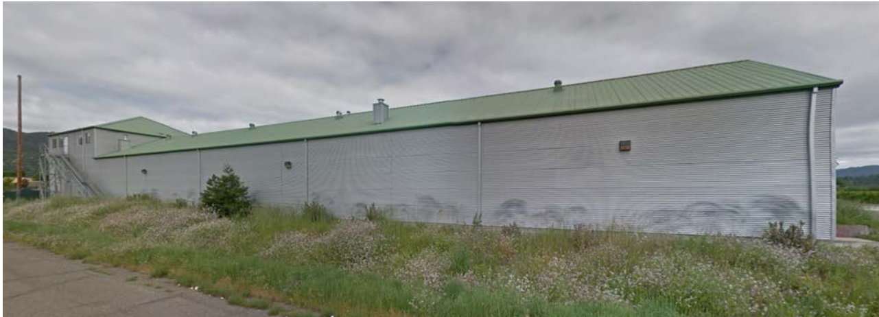
1 SOUTH FACADE FROM HASTINGS RD.
