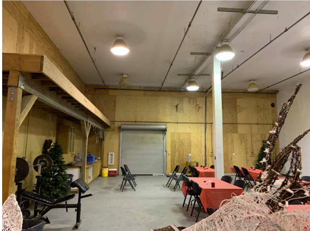
1 EXISTING OPEN AREA UNDER SECOND FLOOR
