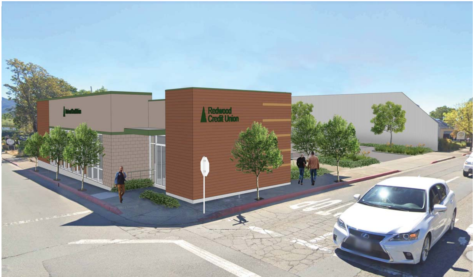
VIEW FACING SOUTH- EAST
