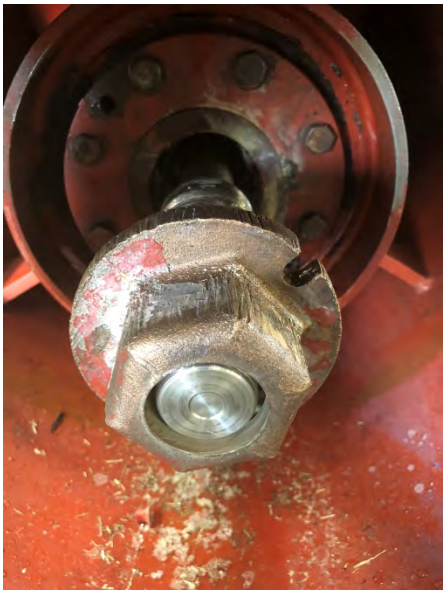
Picture #5 – Picture after removal. Bearing surface will be replaced. Overall this is in good condition.
