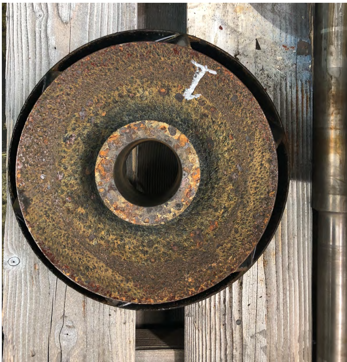
Picture #16 – Impellers are to be reused with reconditioning. The reconditioning will be a steam clan and wire brush to remove deposits and scale.
