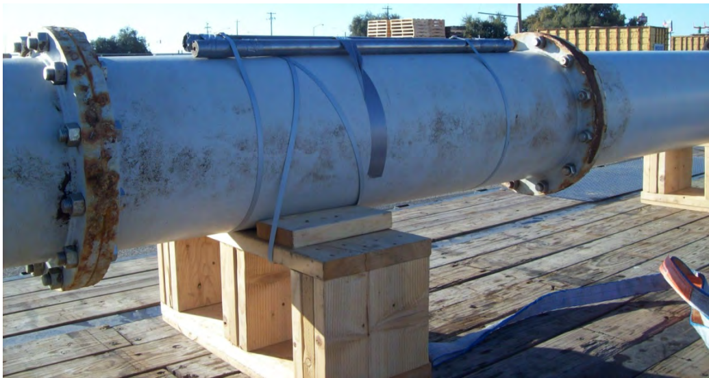
Picture #1 – Pump was received on a flatbed in good condition. Head shafts were received with the units.
