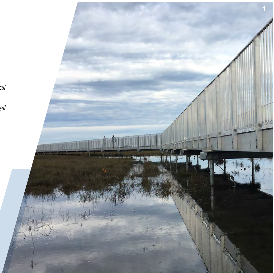
3 Site of Orick Levee Trail, Eureka, CA
