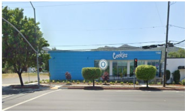
Figures 4 and 5: Photos of the Existing Building
