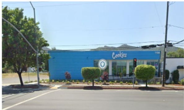
Figures 4 and 5: Photos of the Existing Building
