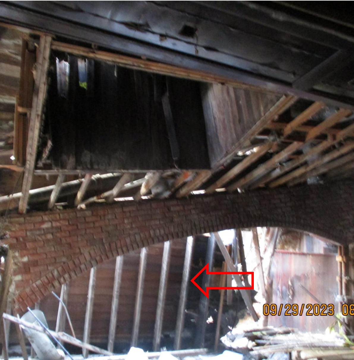
ROOF FROM APOVE 2ND FLOOR
