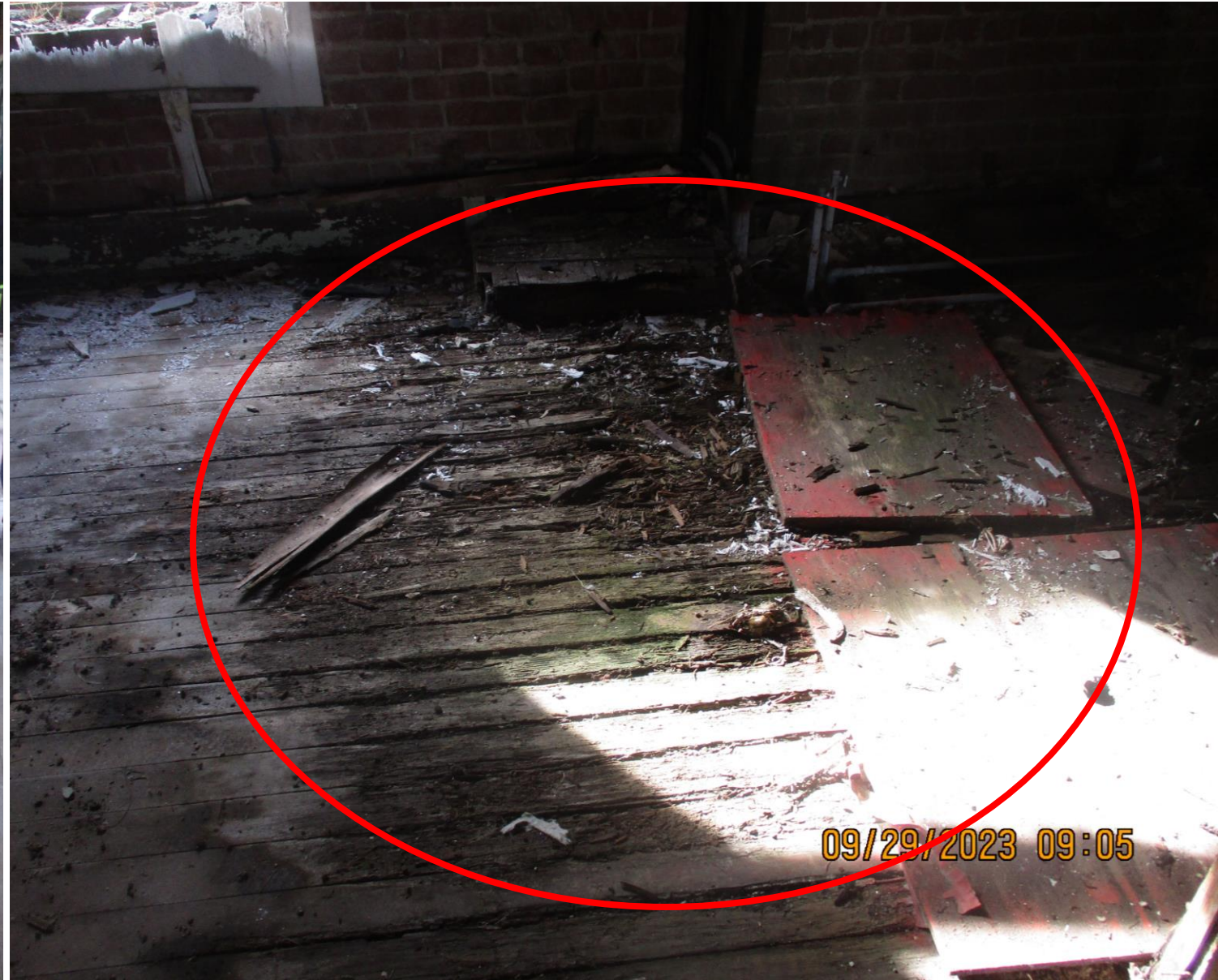
2 ND FLOOR UNEVEN AND COMPROMISED, SMITH ST SIDE. DRY-ROT FLOOR ALSO COMPROMISED
