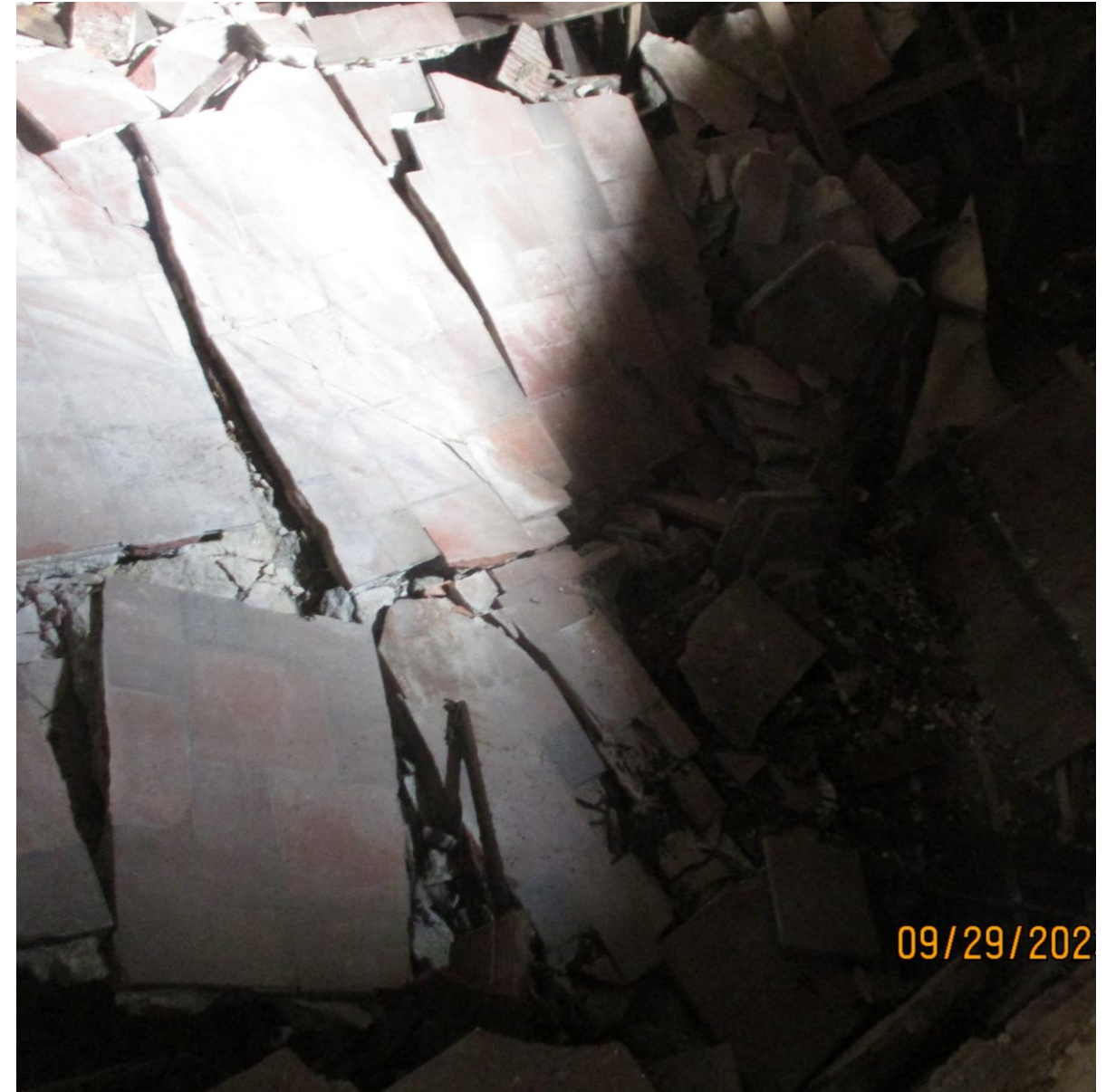
1 ST FLOOR LOOKING AT 1 ST FLOOR, AT STATE ST SIDE OF BUILDING. FLOOR JOIST STRUCTURAL FAILURE
