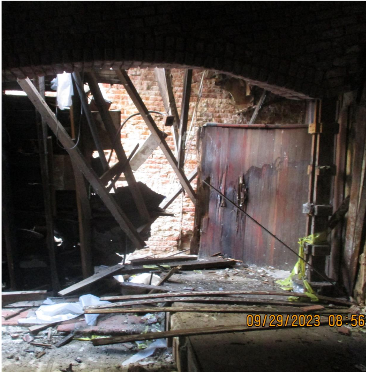
1 ST FLOOR: 2 ND FLOOR STRUCTURAL FAILURE
