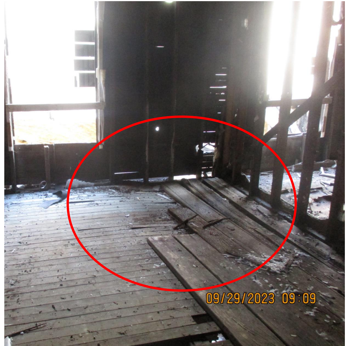
2 ND FLOOR UNEVEN AND COMPROMISED, SMITH ST SIDE. DRY-ROT FLOOR ALSO COMPROMISED, STRUCTURAL FAILURE
