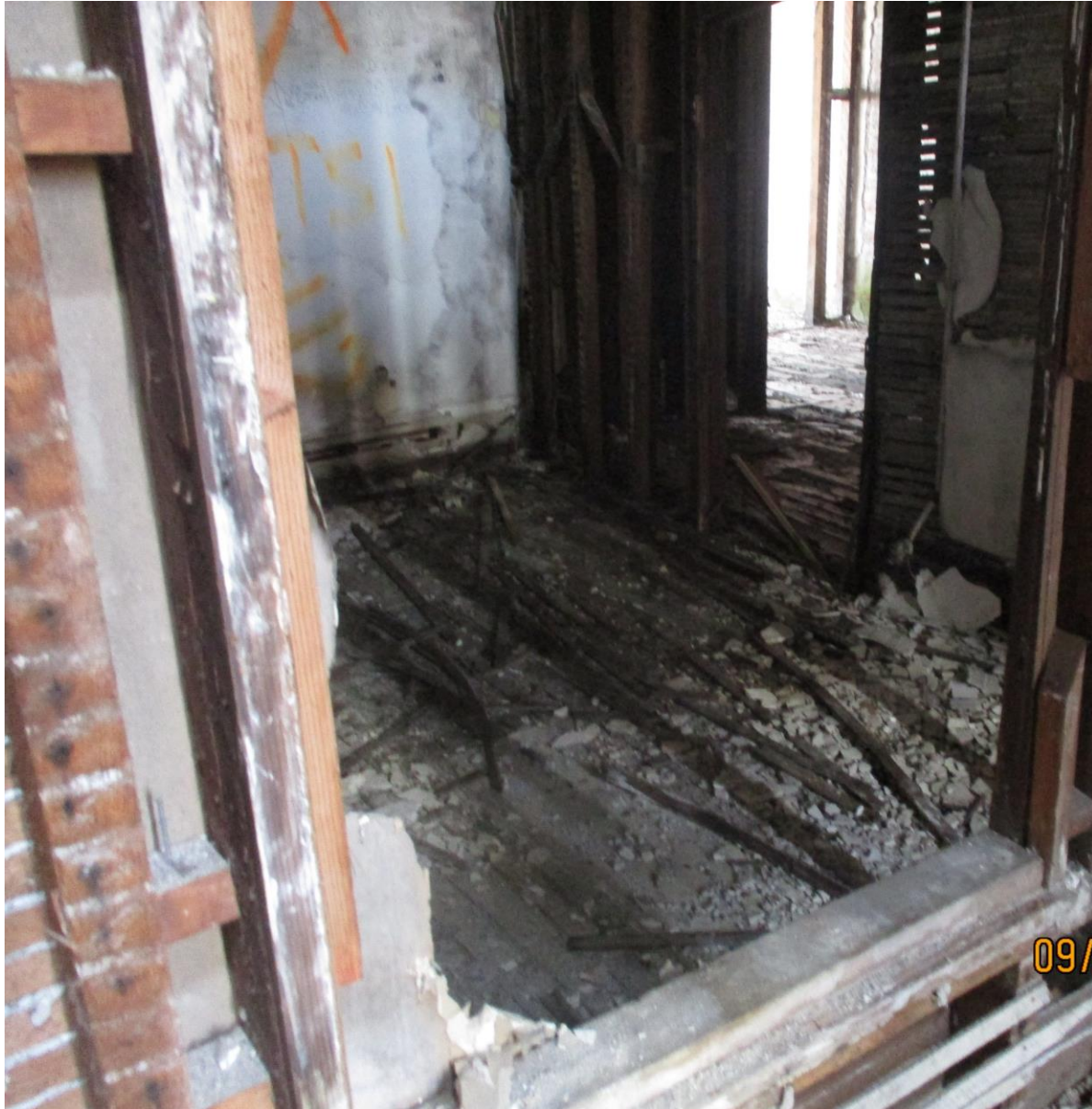
2 ND FLOOR FIRE HAZARD EXPOSED WOOD
