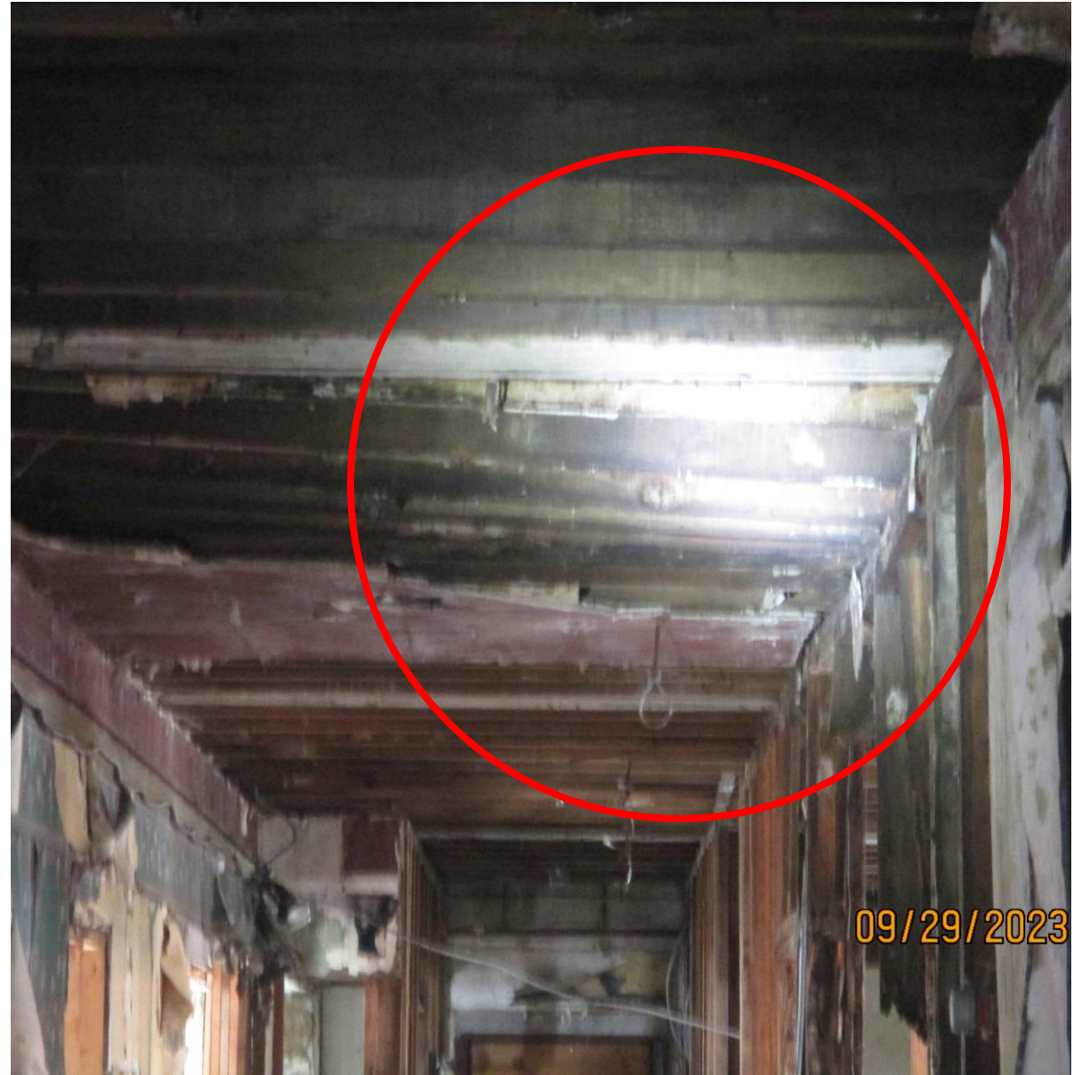
2nd FLOOR LOOKING AT 3rd FLOOR. FLOOR JOIST STRUCTURAL FAILURE
