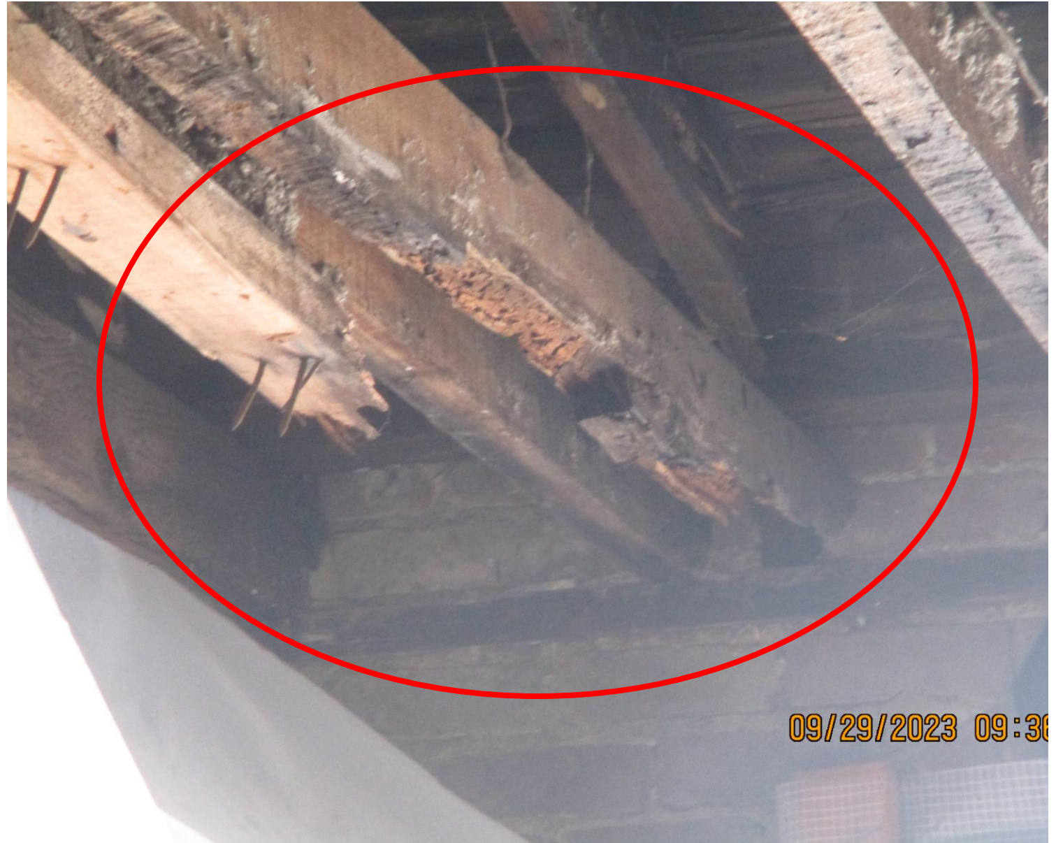
3 RD FLOOR UNEVEN AND COMPROMISED, SMITH ST SIDE. DRY-ROT FLOOR ALSO COMPROMISED, STRUCTURAL FAILURE
