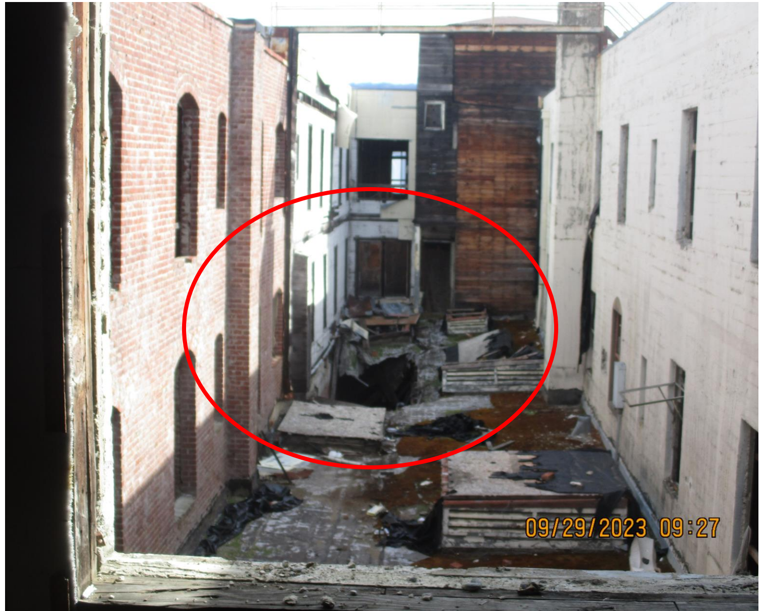
3 rd FLOOR LOOKING AT 2 ND FLOOR ATRIUM. FLOOR JOIST/ROOF STRUCTURAL FAILURE
