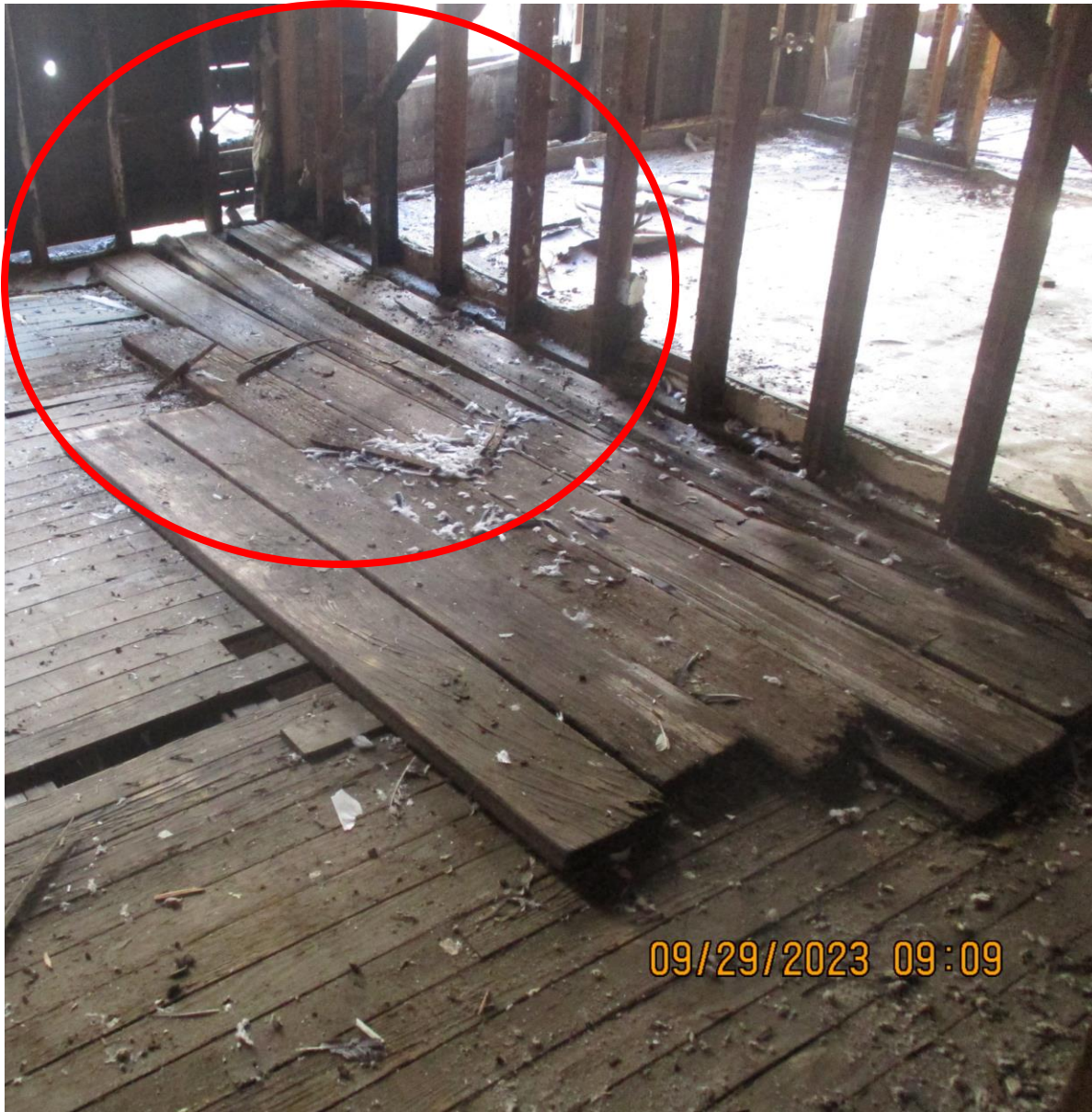
2 ND FLOOR UNEVEN AND COMPROMISED, SMITH ST SIDE. DRY-ROT FLOOR ALSO COMPROMISED, STRUCTURAL FAILURE
