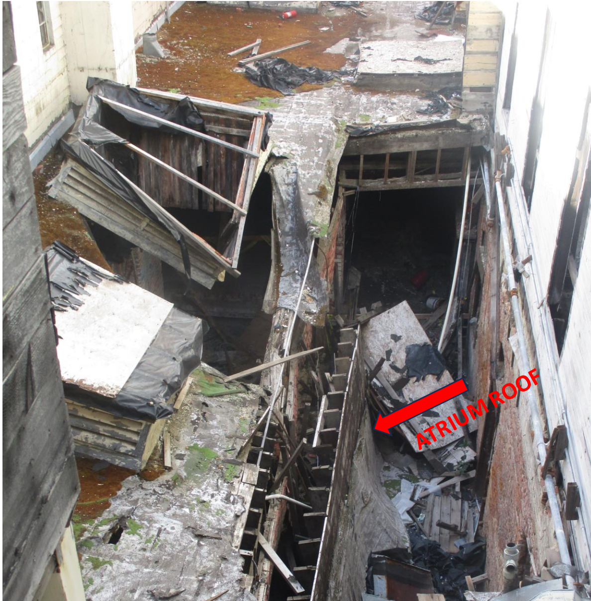
3RD FLOOR COLLAPSED ATRIUM FROM ABOVE
