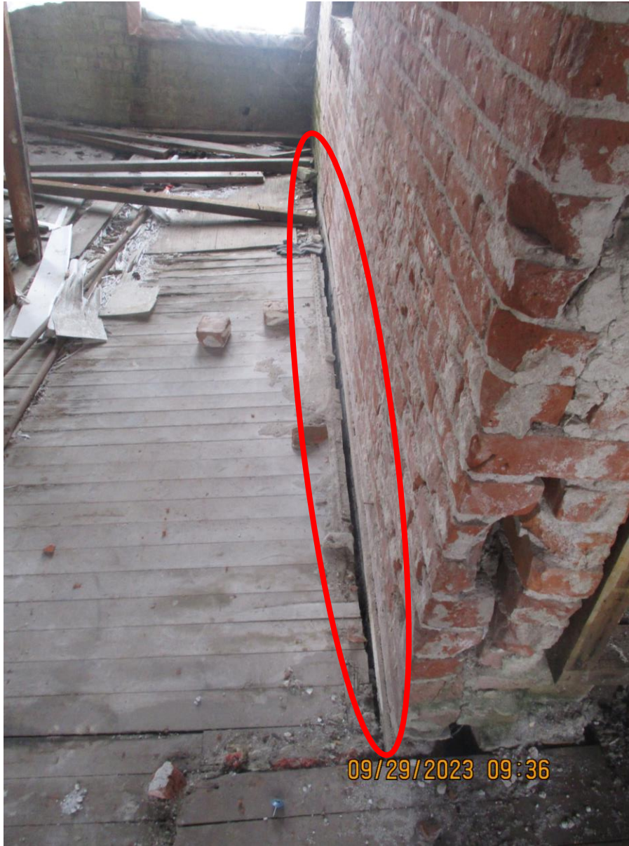
3 RD FLOOR UNEVEN AND COMPROMISED, SMITH ST SIDE. DRY-ROT FLOOR ALSO COMPROMISED, STRUCTURAL FAILURE
