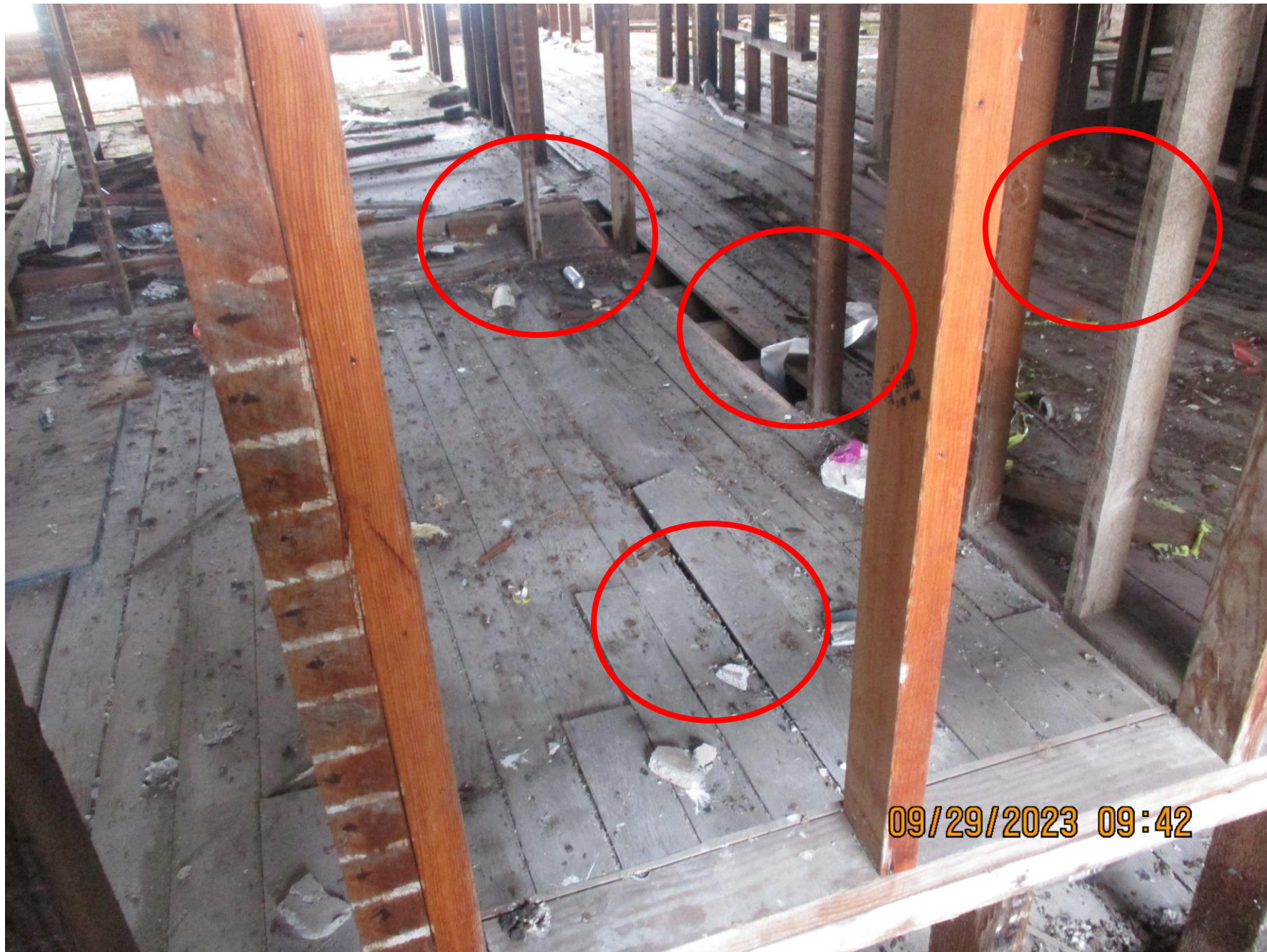
3 RD FLOOR UNEVEN AND COMPROMISED, STATE. DRY-ROT FLOOR ALSO COMPROMISED, STRUCTURAL FAILURE
