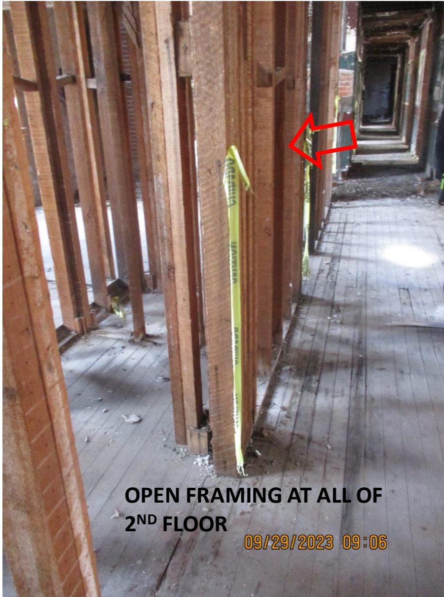
2 ND FLOOR UNEVEN AND COMPROMISED, SMITH ST SIDE. DRY-ROT FLOOR ALSO COMPROMISED
