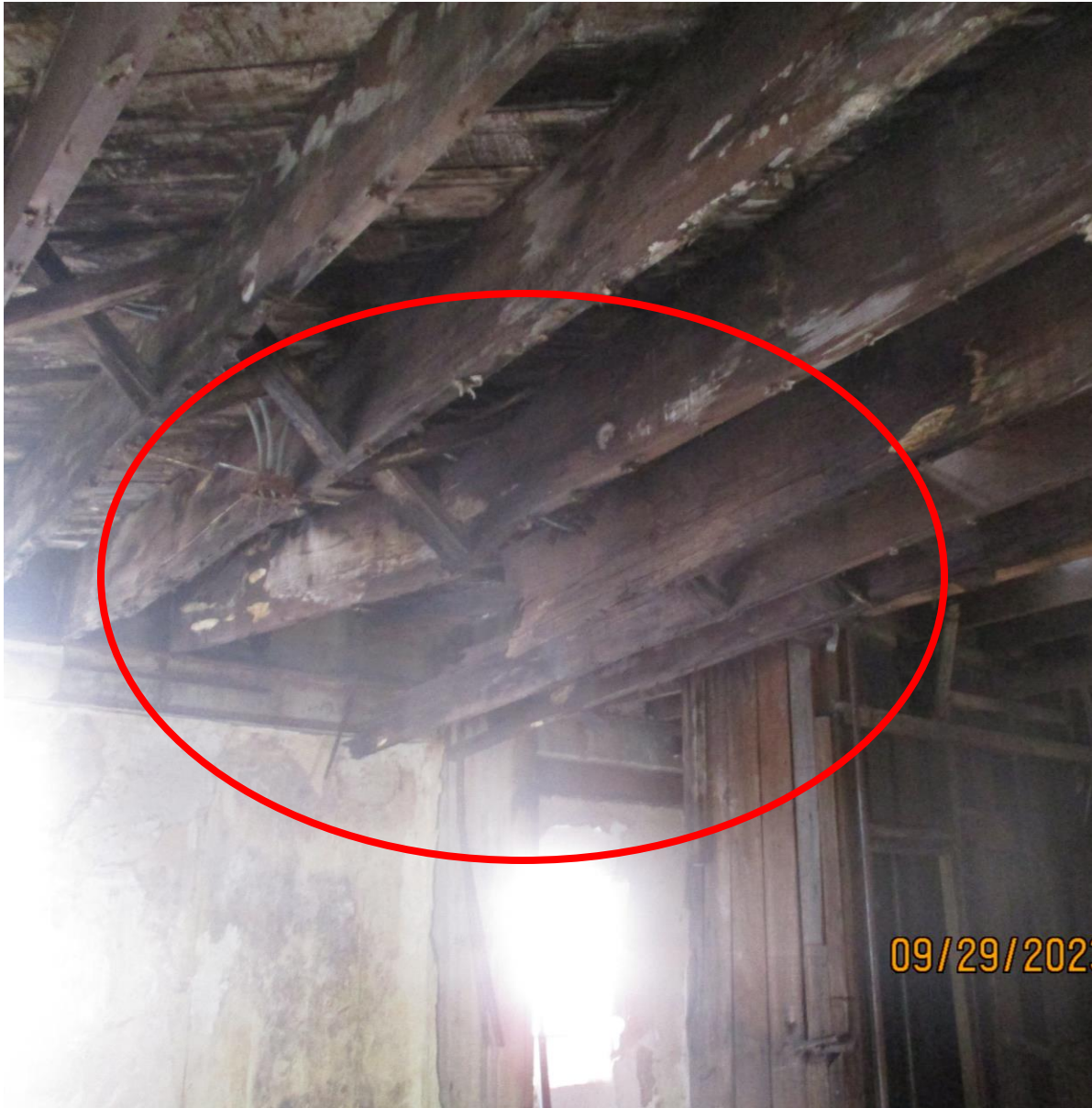
2nd FLOOR LOOKING AT 3rd FLOOR. FLOOR JOIST STRUCTURAL FAILURE
