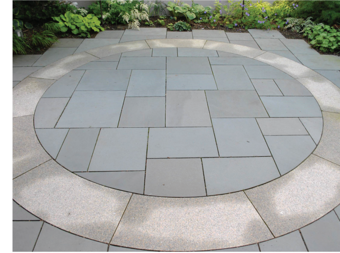
Bluestone pavers with concrete band
