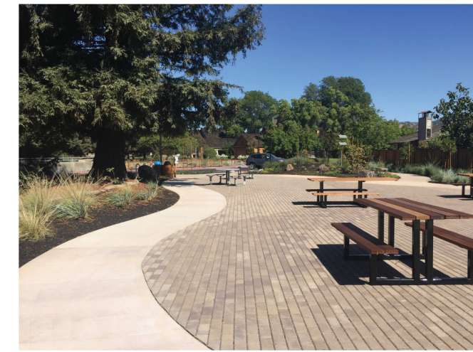
Integrally colored concrete path and permeable paving
