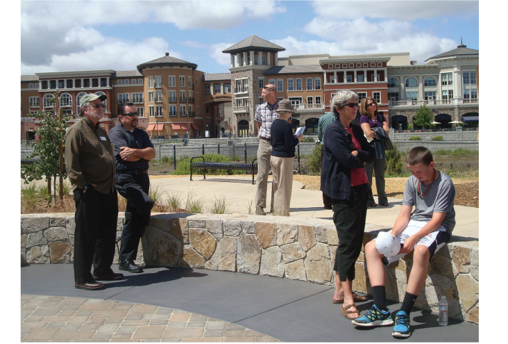
Concrete pavers, integrally colored concrete and stone seat wall
