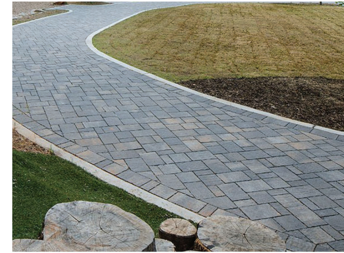
Permeable paver path with concrete edge
