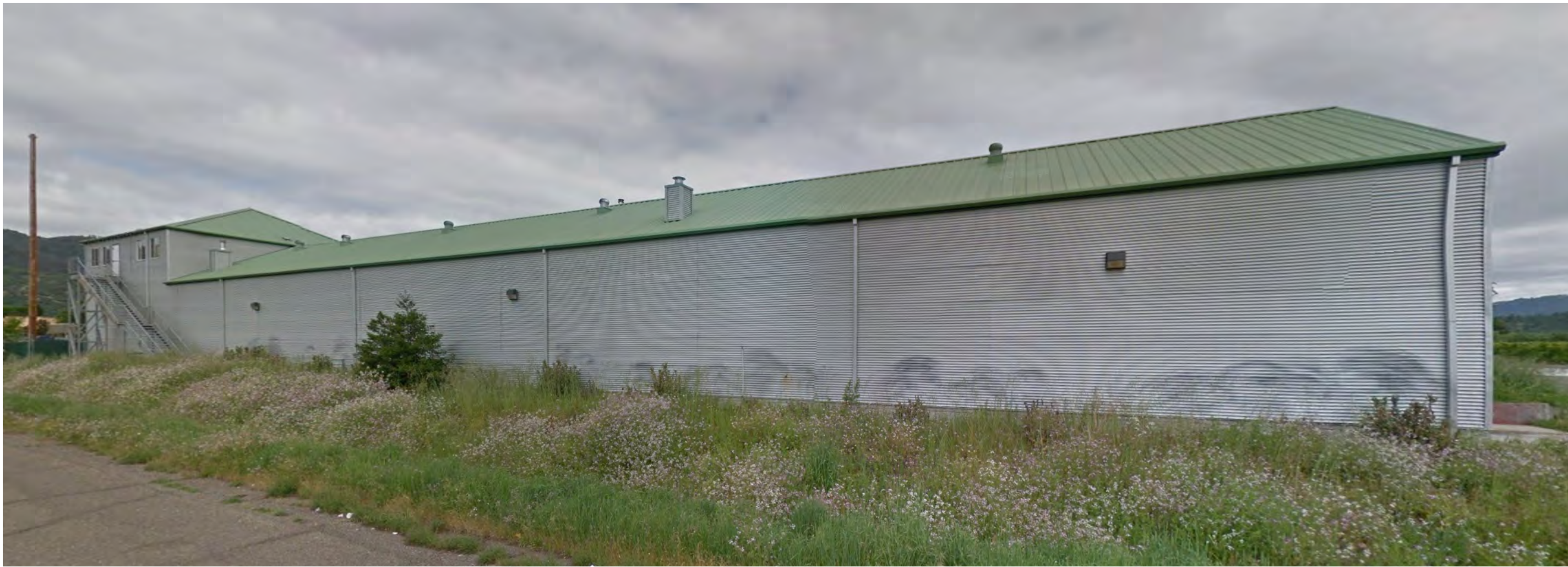
1 SOUTH FACADE FROM HASTINGS RD.
