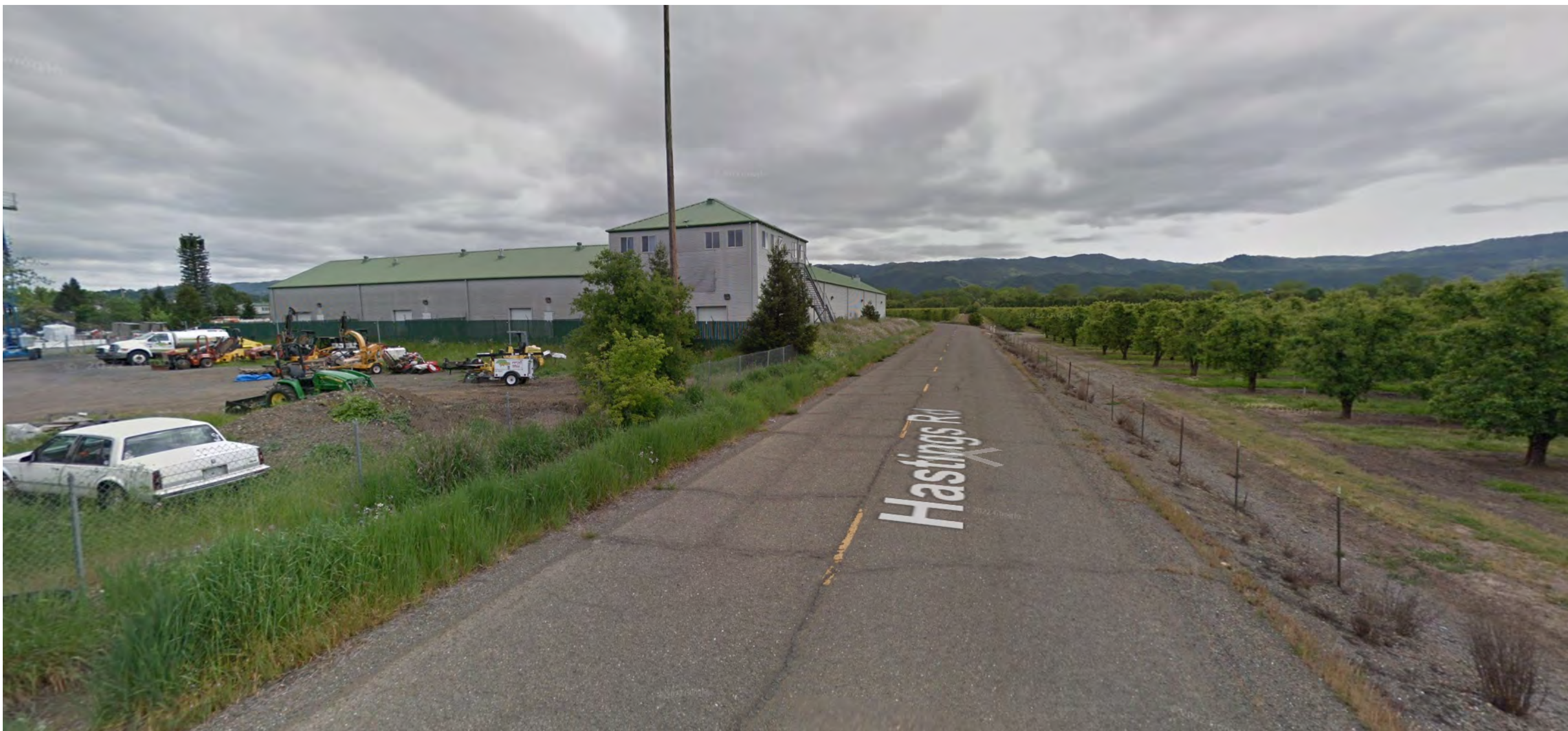
3 WEST FACADE FROM HASTINGS RD.
