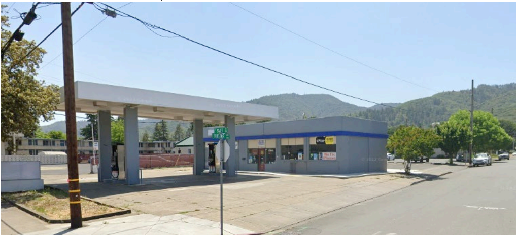
View via Freitas Avenue, front
