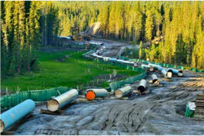
Laying out the Trans Mountain oil pipeline near Hinton Alberta Canada PHOTO: Robert McGuey / Industry / Alamy Stock Photo
