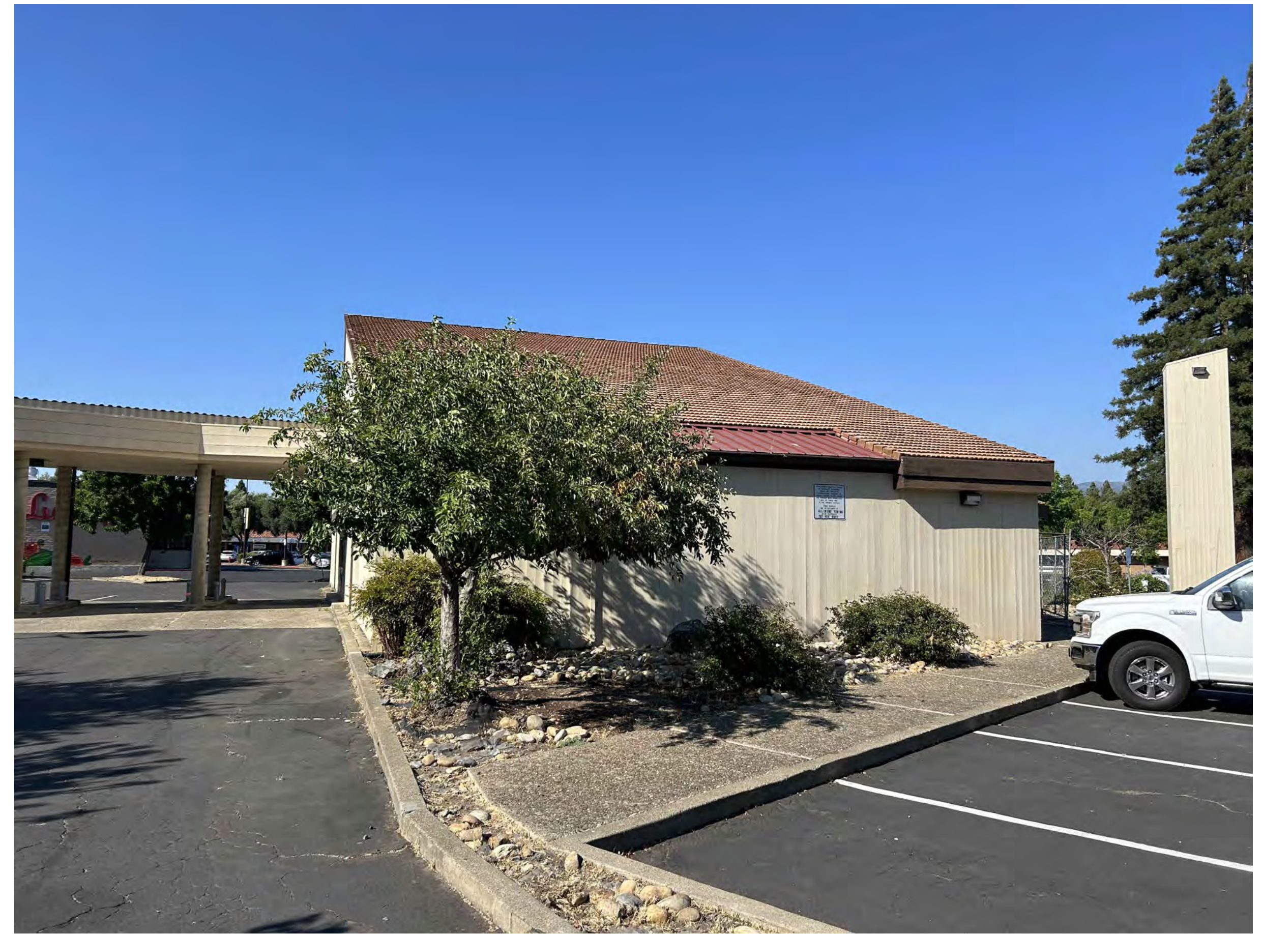
(FRONT WALL; SOUTH SIDE)
