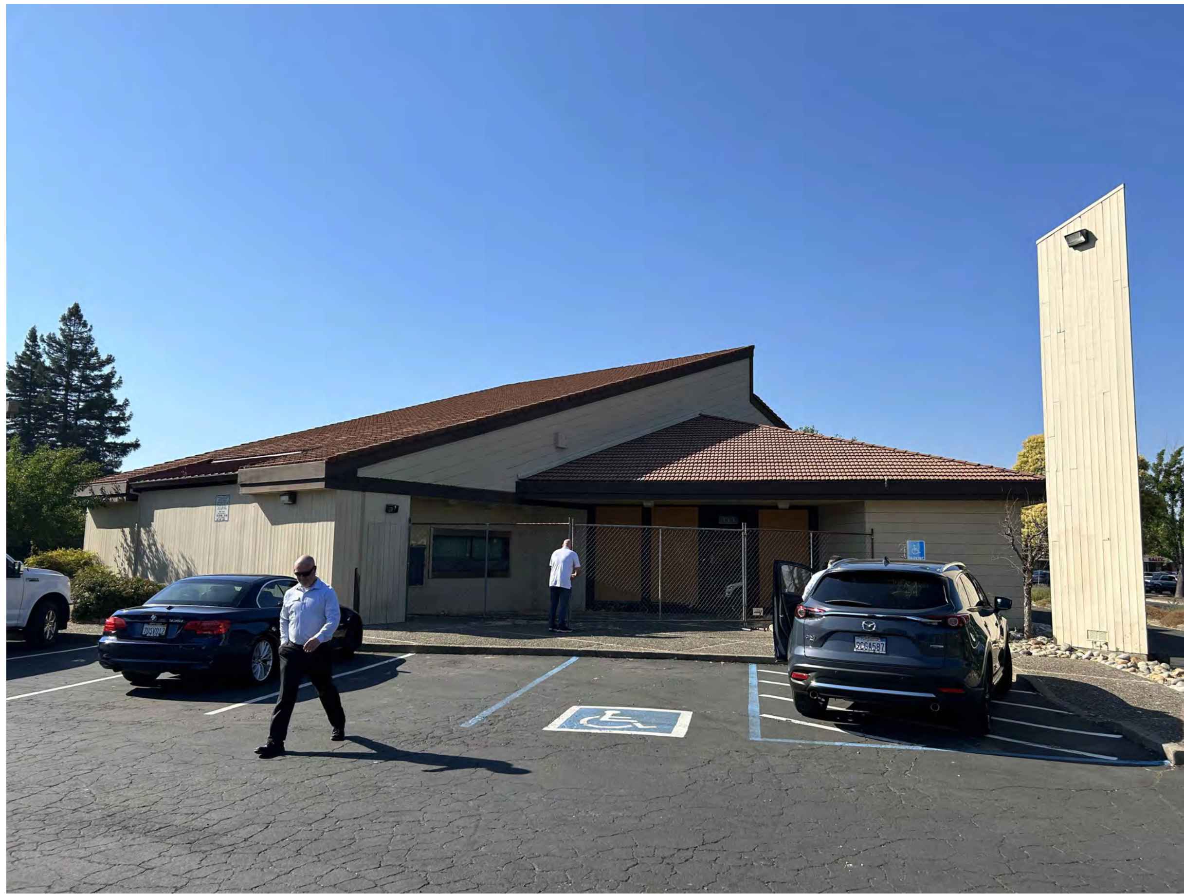
(FRONT ENTRY; SOUTH SIDE)
