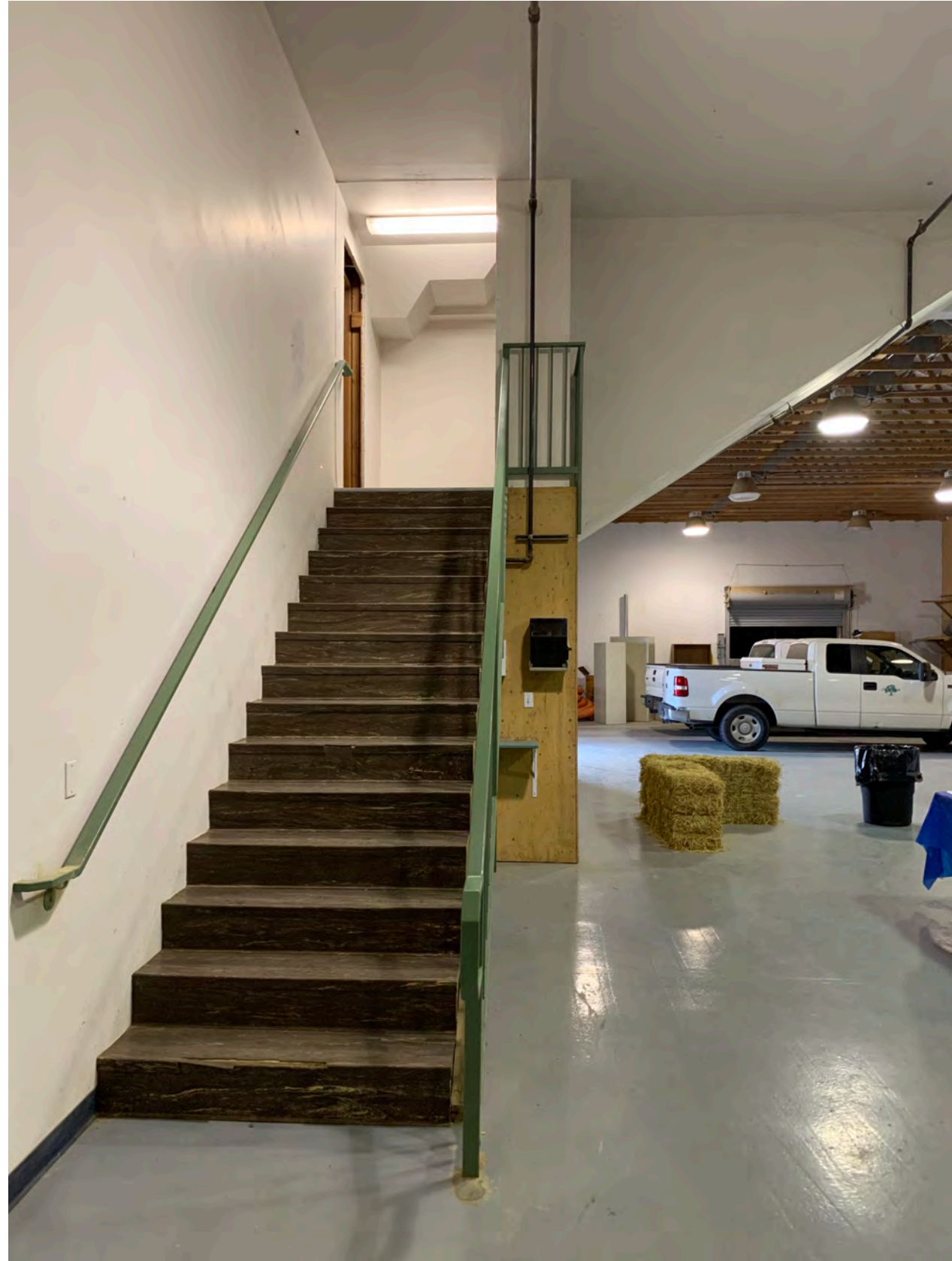
6 EXISTING STAIR TO SECOND LEVEL
