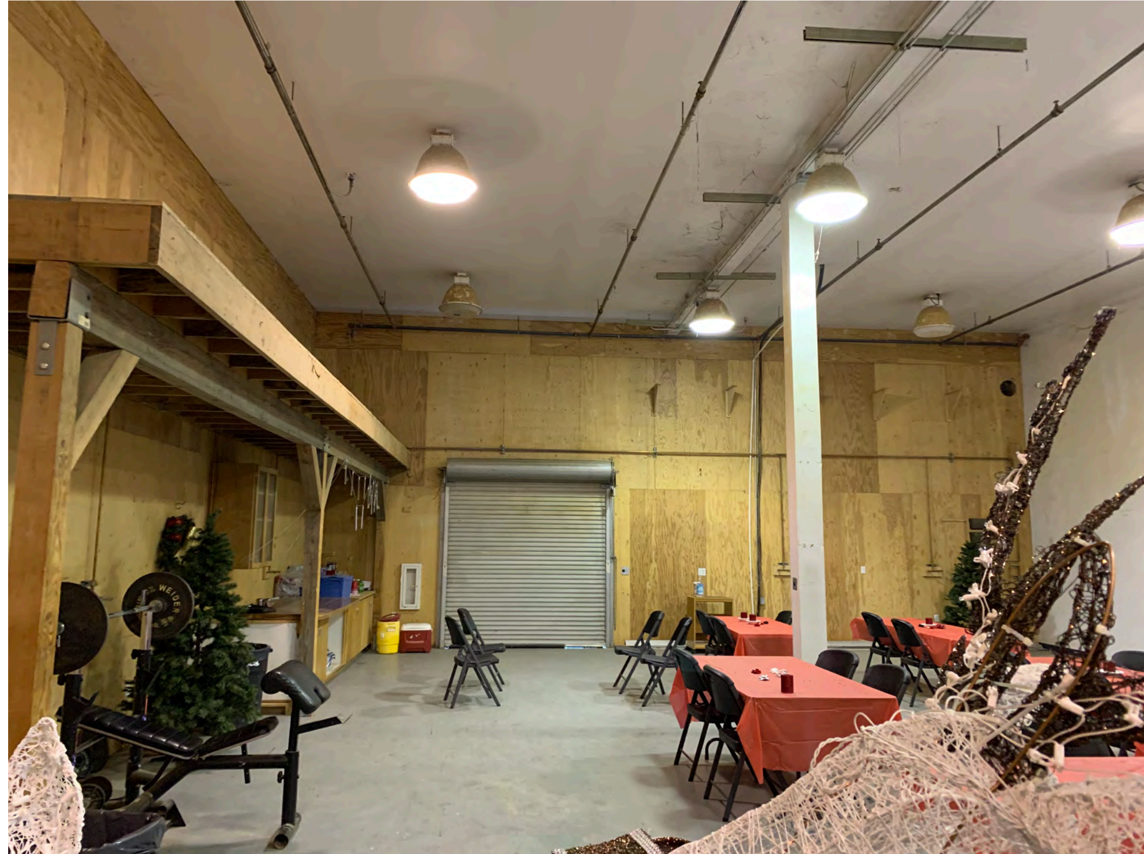
1 EXISTING OPEN AREA UNDER SECOND FLOOR
