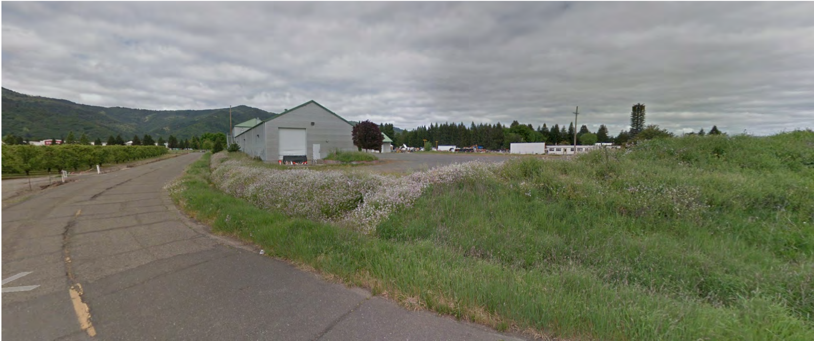
2 EAST FACADE FROM HASTINGS RD
