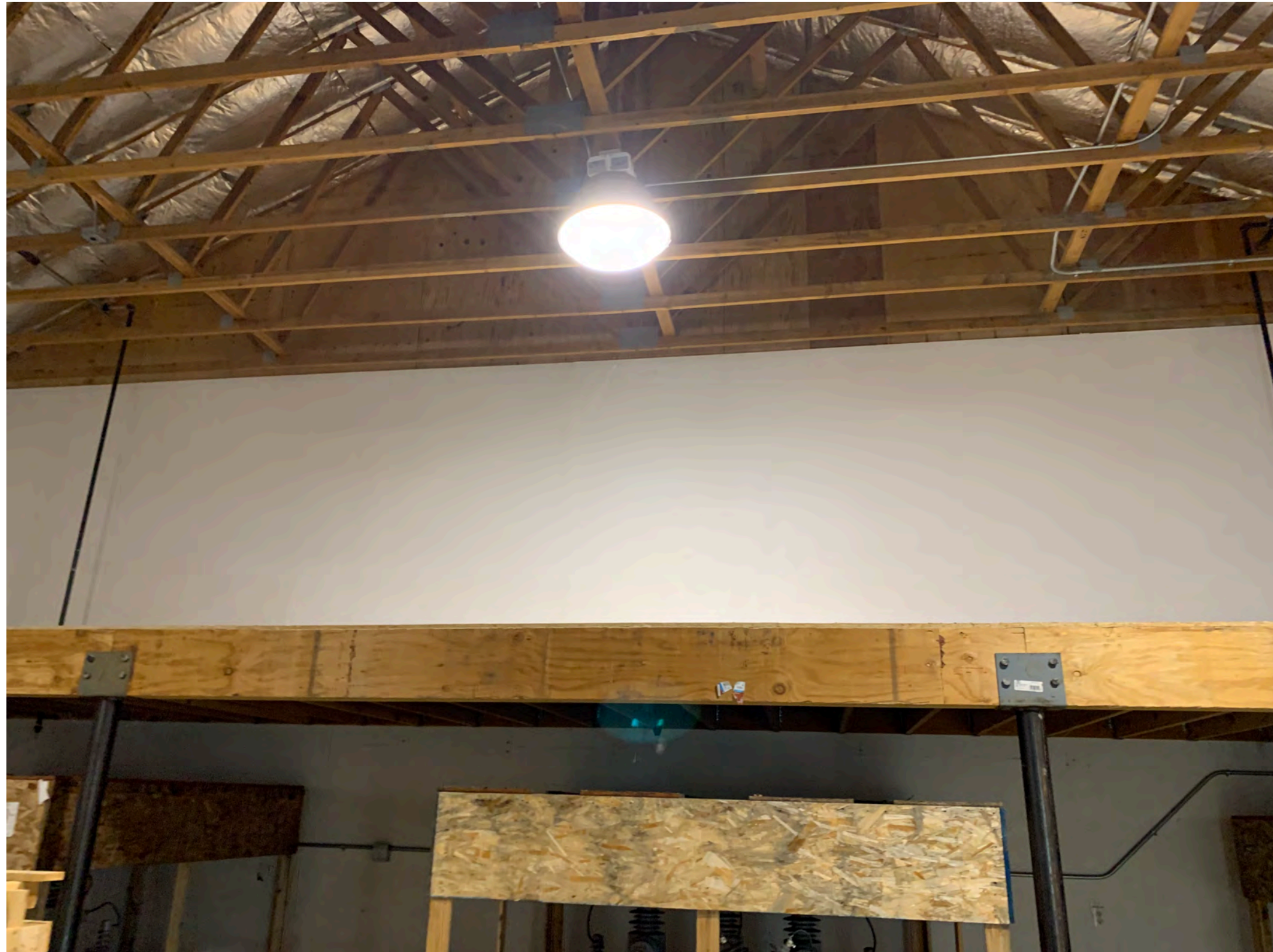
5 EXISTING BAY 2 MEZZANINE
