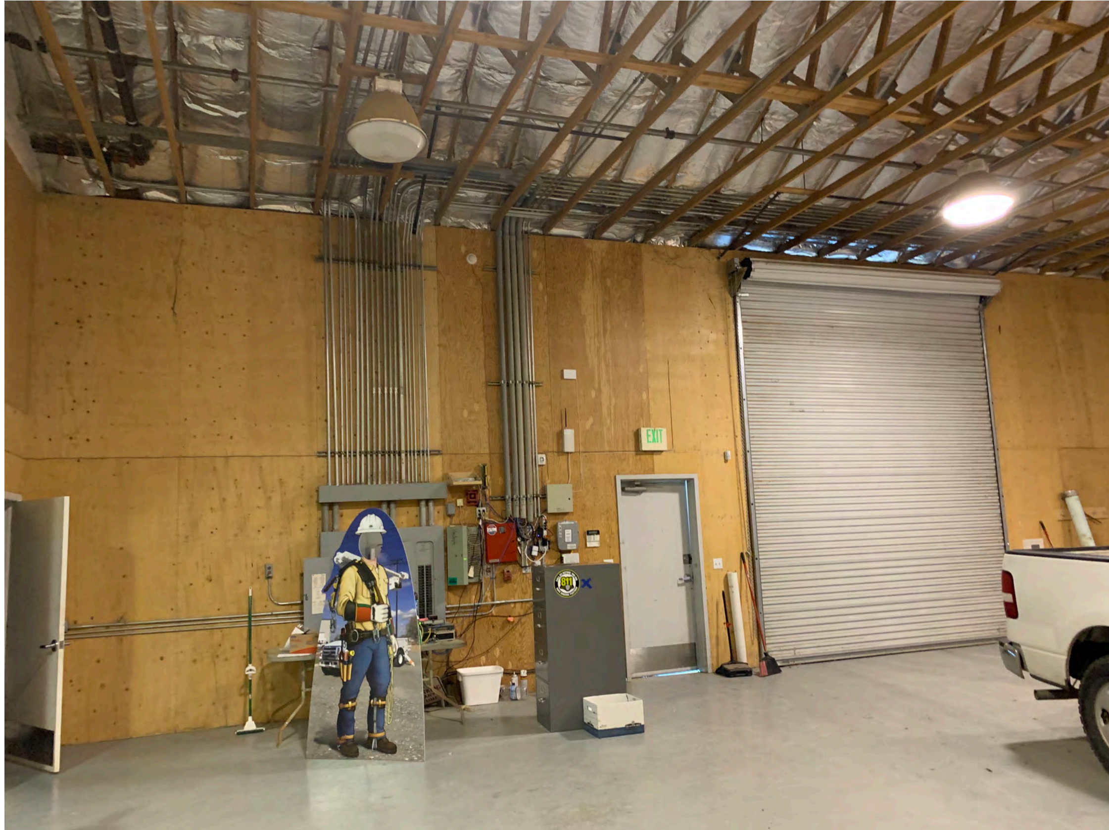
2 EXISTING READY ROOM AREA / MECH. RM.
