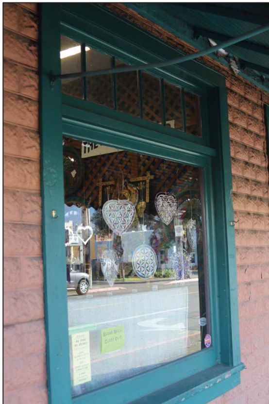
Photo 32: West elevation, window with multi lite transom (original)
