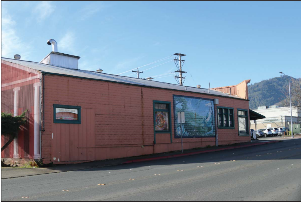
Photo 45: North elevation (fronting Perkins Street)
