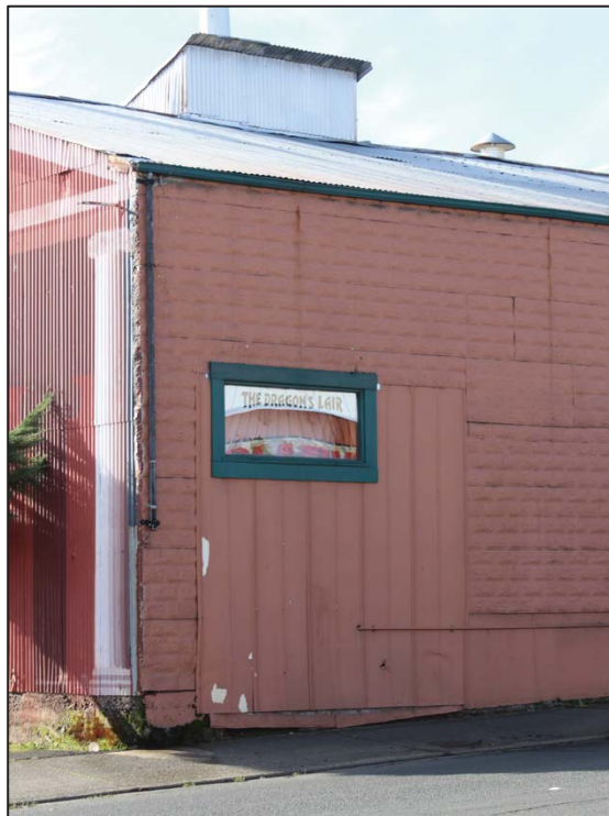
Photo 46: North elevation, infilled bay at NE corner
