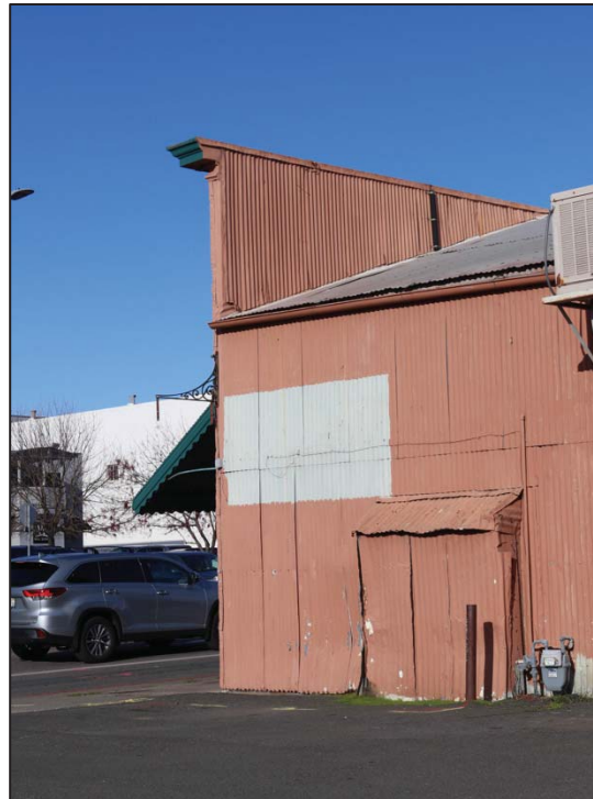
Photo 38: West elevation false front (looking NW)
