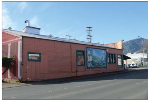
North Elevation (Perkins Street)
