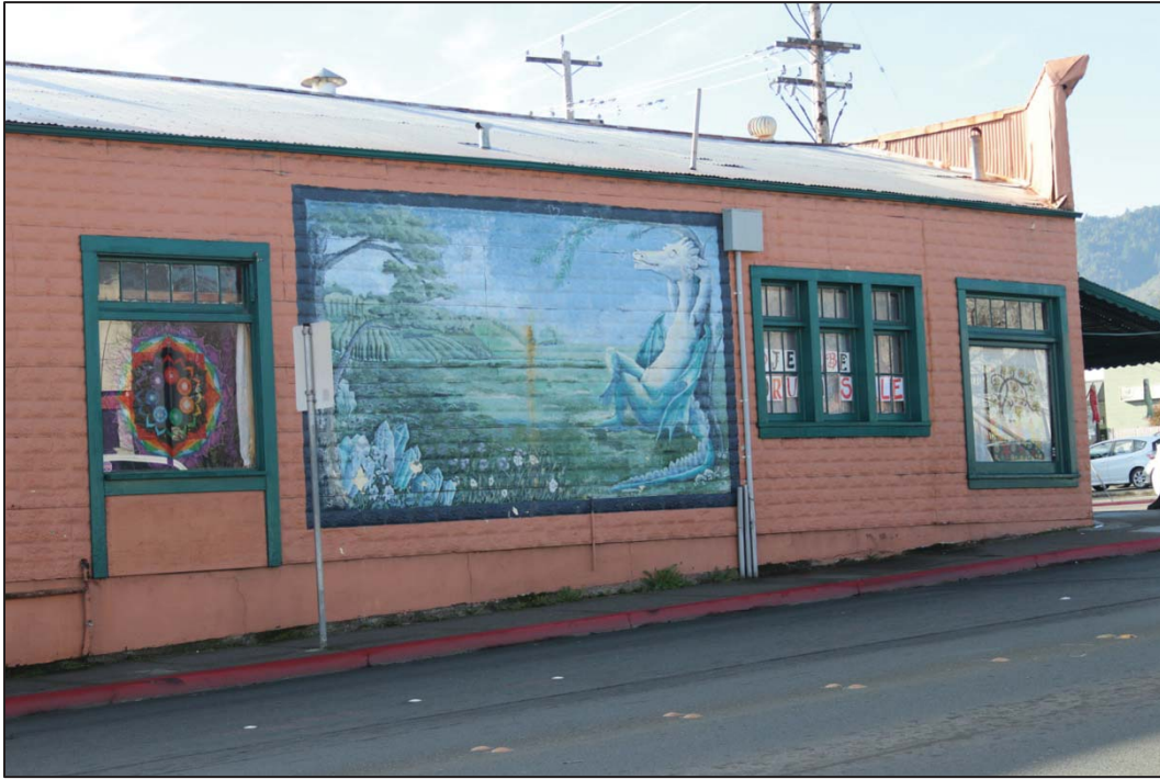
Photo 47: North elevation, mural and windows
