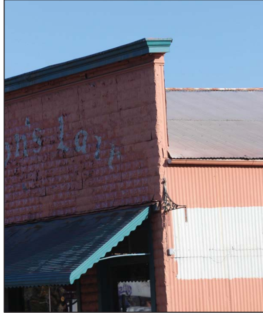
Photo 37: West elevation, false fronting (looking NE)
