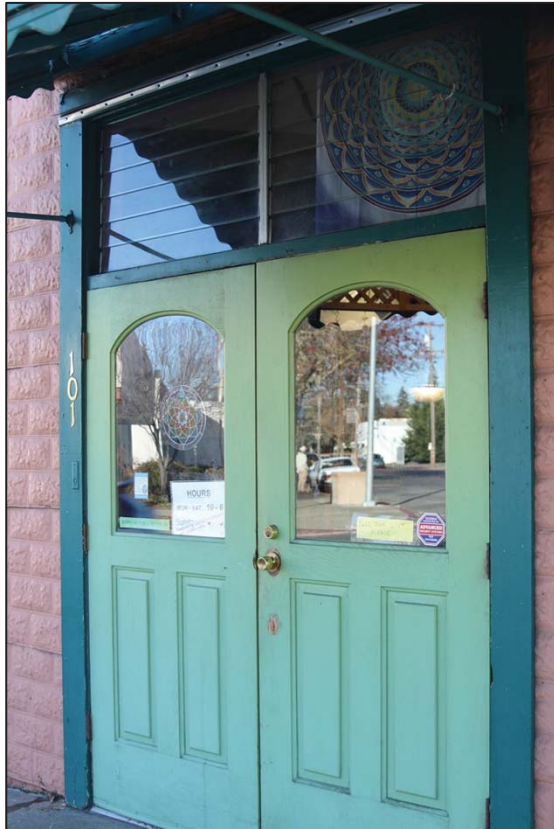
Photo 30: Northwest corner, door and jalousie transom (not original)
