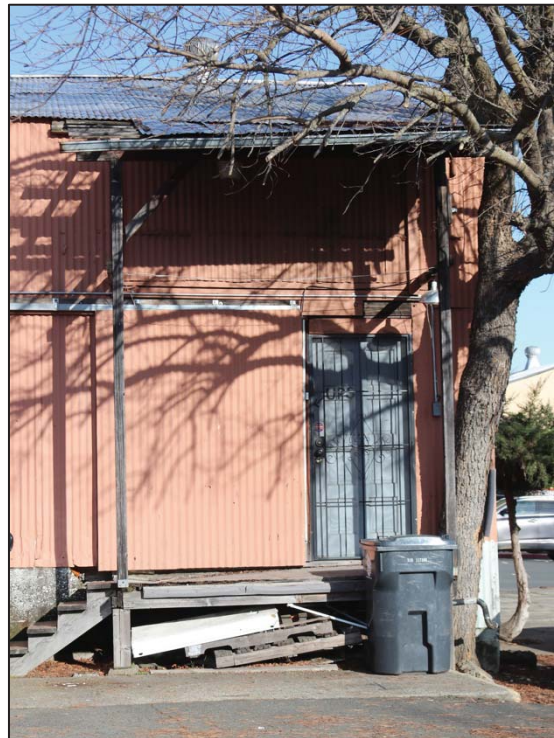
Photo 42: South elevation, pedestrian entrance at SE corner
