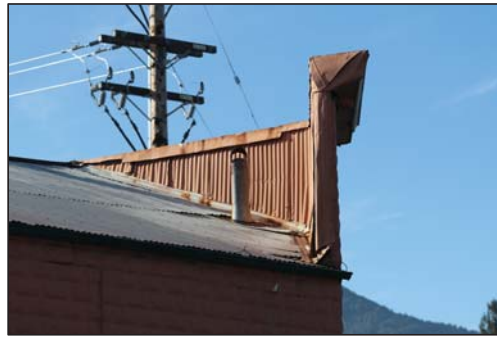
Northwest corner, False Front Detail
