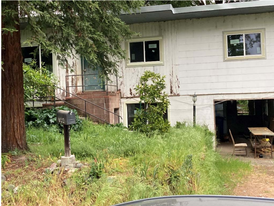
Photo #4: Single-family home, possibly vacant due to hazards
