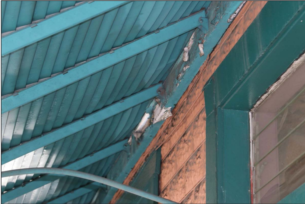
Photo 35: West elevation, ceiling of awning
