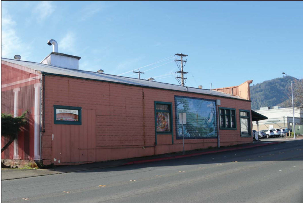
Photo 45: North elevation (fronting Perkins Street)
