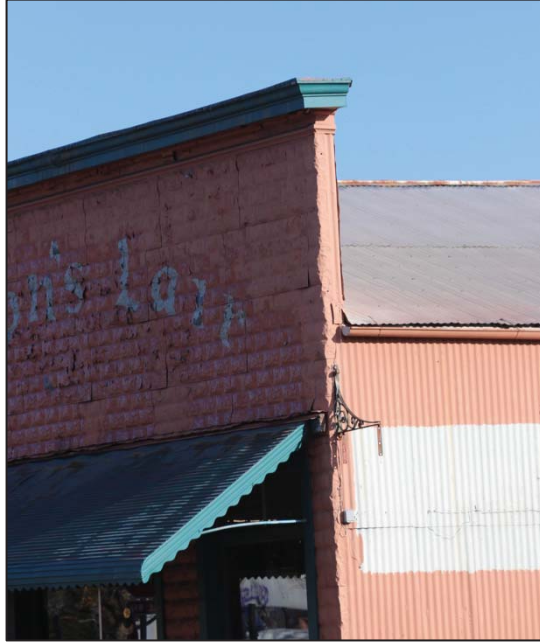
Photo 37: West elevation, false fronting (looking NE)
