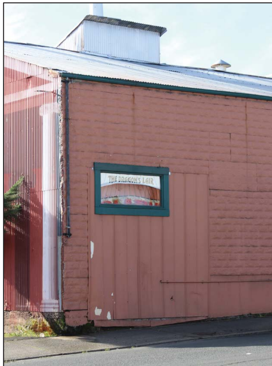
Photo 46: North elevation, infilled bay at NE corner
