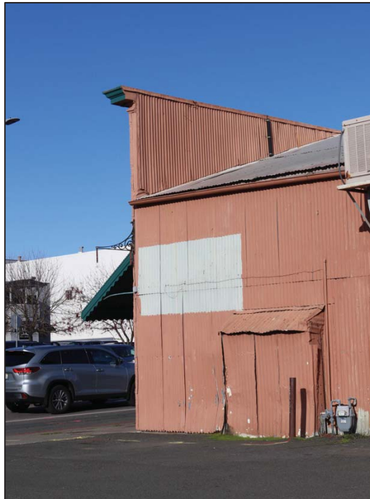
Photo 38: West elevation false front (looking NW)
