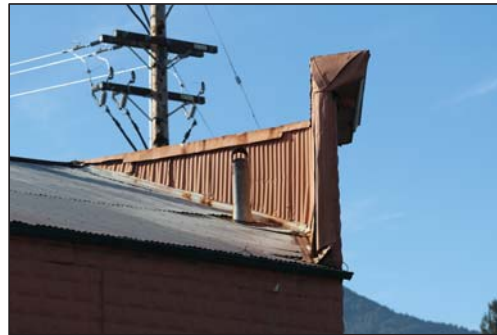
Northwest corner, False Front Detail
