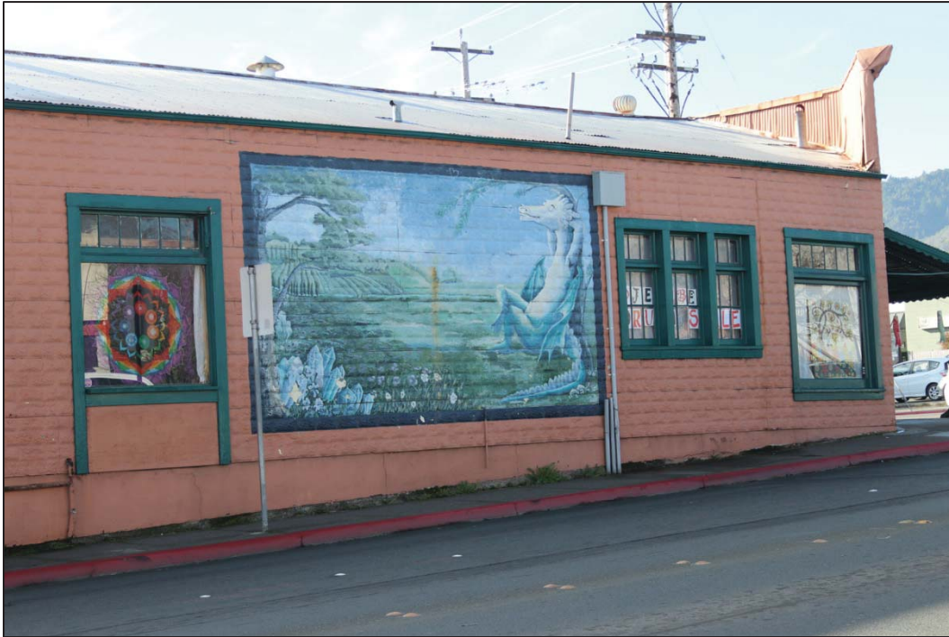
Photo 47: North elevation, mural and windows
