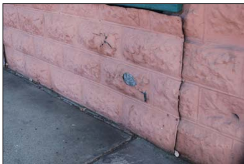
West Elevation, Pressed Tin Detail
