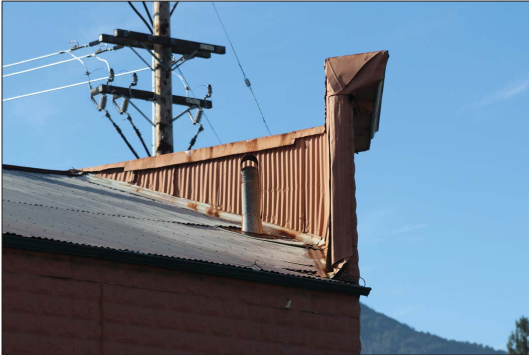
Photo 39: West elevation, false front (looking SW)
