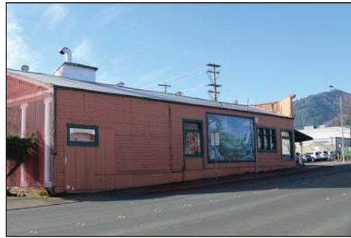
North Elevation (Perkins Street)
