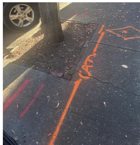
Utility markings in conflict with the tree.
