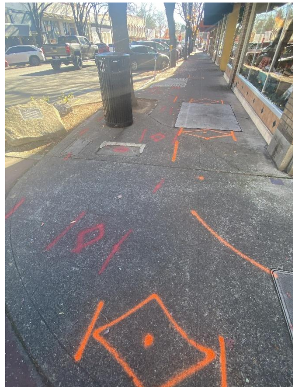
811 Utilities Marking, Ukiah, CA.
