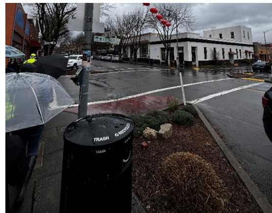
Informal extension of the curb at Church Street.
