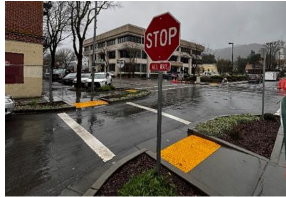
Curb extensions across Smith Street.
