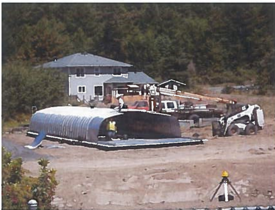
Assembly of arch culvert (Phase 1).
