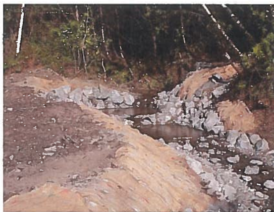
Restored stream channel (Phase 2).
