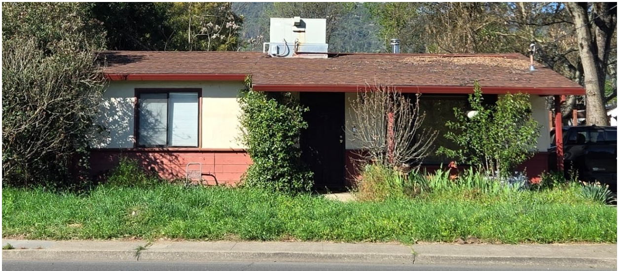
Example: Housing Unit in a Condition of Substantial Deterioration
