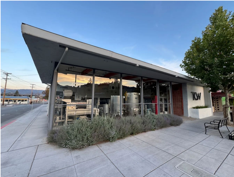
401 S State Street – Post-Adaptive Reuse (TCW)
