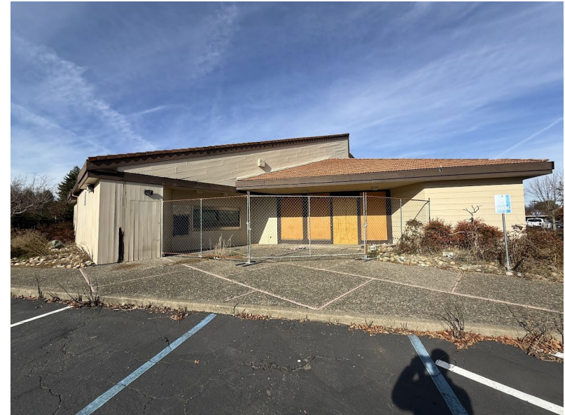
414 East Perkins Street- Pre-Adaptive Reuse (RCU)
