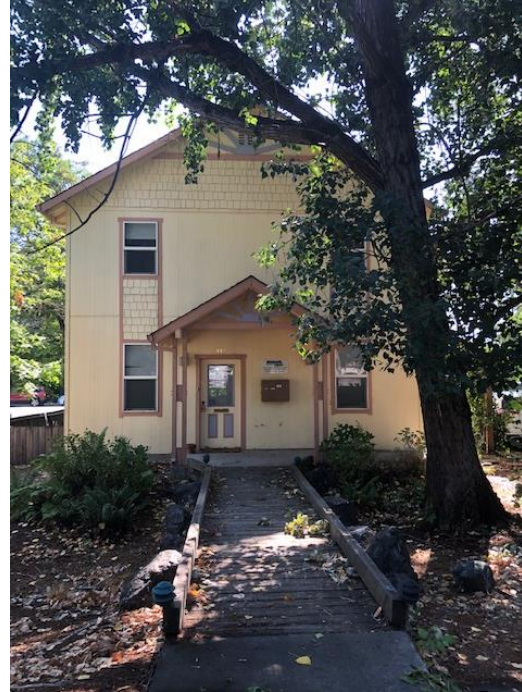
Figure 5: North State Street frontage
