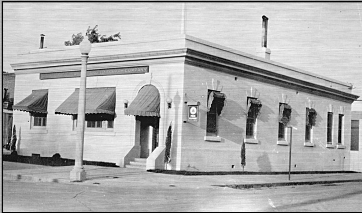
March 2, 1917 - Pacific Telephone and Telegraph Company Building at Church and School Streets; new Home of Ukiah's "Hello Girls"
